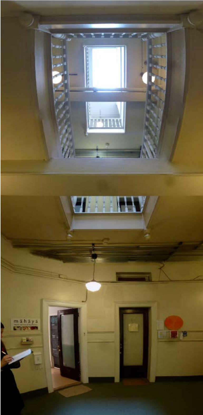
View of light well from ground floor.
