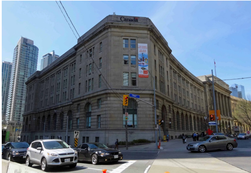
Exterior photograph, showing the Dominion Public Building at the southwest corner of Front Street West and Yonge Street (Heritage Preservation Services, 2015)
