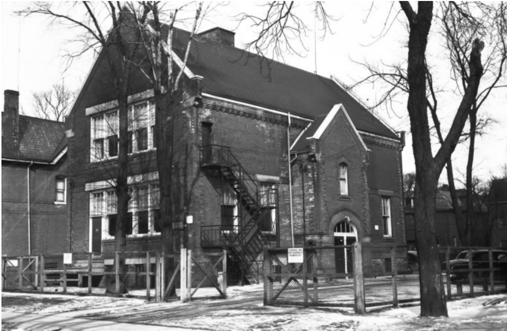
above: archival photograph, 1955, showing the principal (south) elevation of the Allan School (right) and the west wall facing George Street (left) (Toronto Public Library, Item 5678); cover: current photograph, 349 George Street
