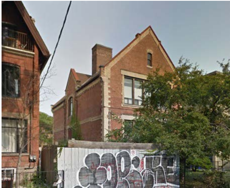
19. Current Photograph, 349 George Street, 2015 : on the left, the rear (north) wall under the cross gable has a shallow frontispiece with window openings, and the decorative brickwork is continued from the adjoining elevations.
