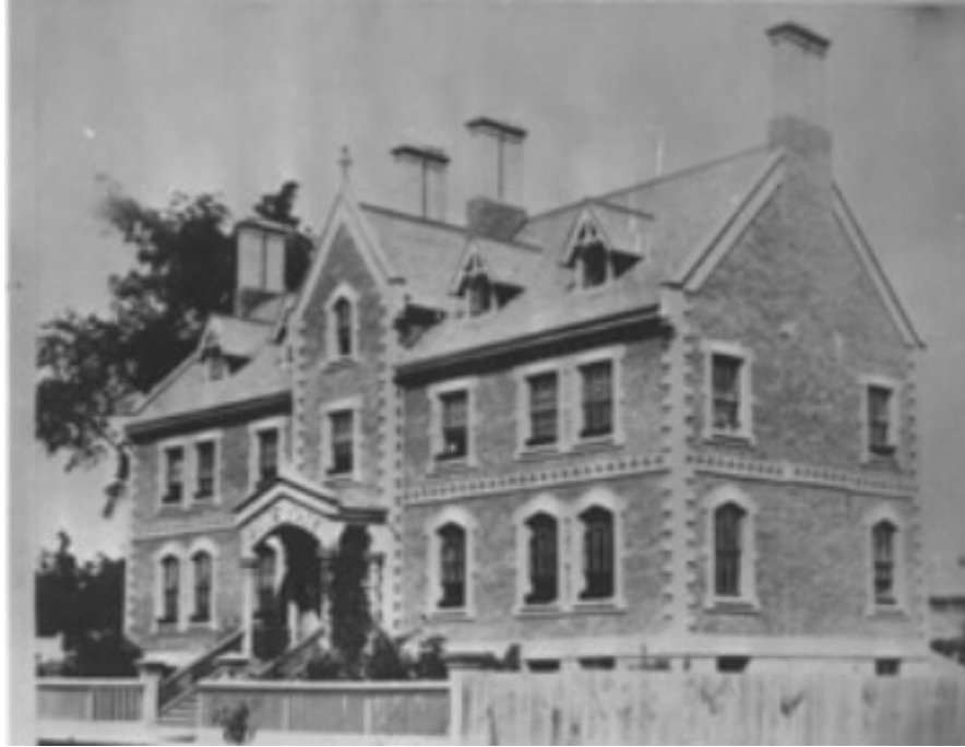
12. Archival Photograph, Toronto Boys Home, 1867 : showing the original building (1864) with the rectangular plan, gable roof with flared eaves, pattern brickwork, and central frontispiece containing the main entrance that are reflected in the design for the Allan School (Toronto Public Library, Item 11781).
