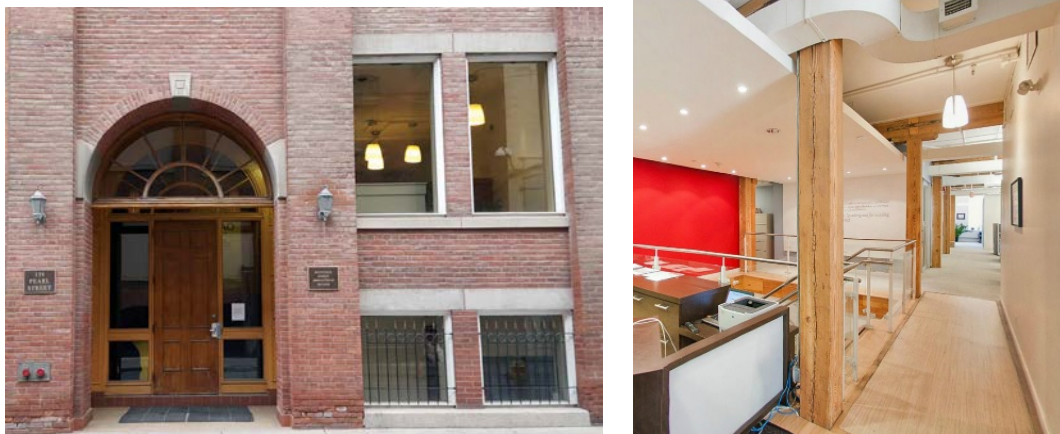
11. Current Photographs, 2015 : showing part of the principal (south) elevation where the entrance was moved to the westernmost bay (left), and the post-and-beam construction exposed on the interior (right) (Heritage Preservation Services and http://tours.willtour360.com/public/vtour/display/39191?a=1 ).
