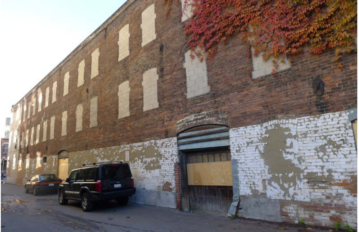
19. Conboy building, west elevation : showing the delivery access openings in the walls, the blocked-in windows and anchor plates. (HPS)
