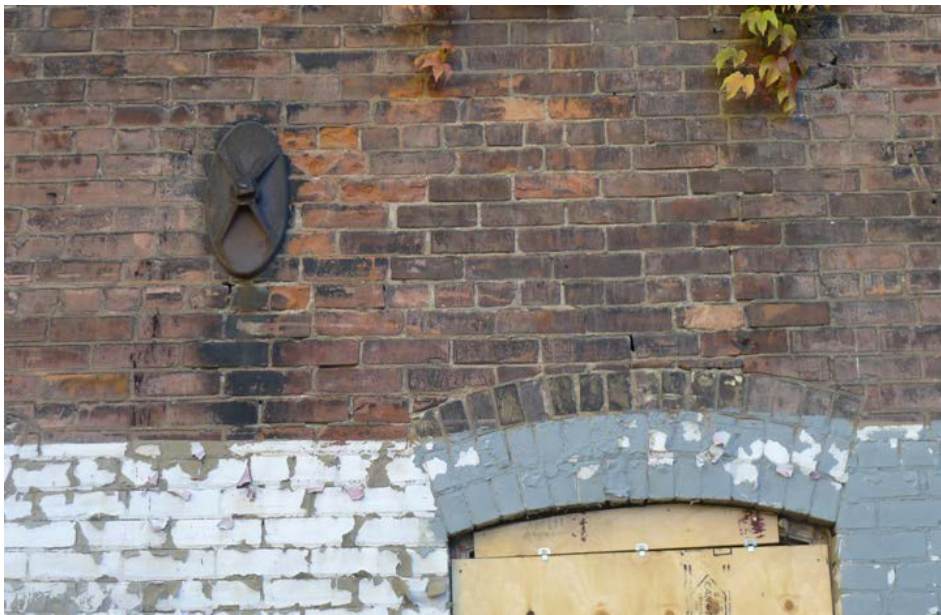
18. Conboy building : showing a detail from the west elevation with brick work, window headers and a cast-iron anchor plate . (HPS)
