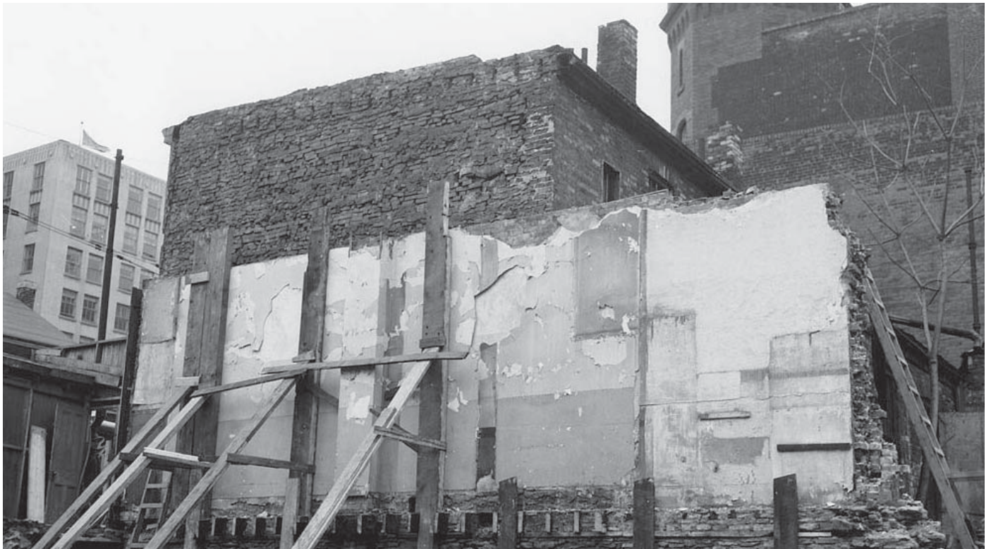
(Above) Building wall being supported during an excavation as part of the Yonge subway line construction, photo taken in 1952.
