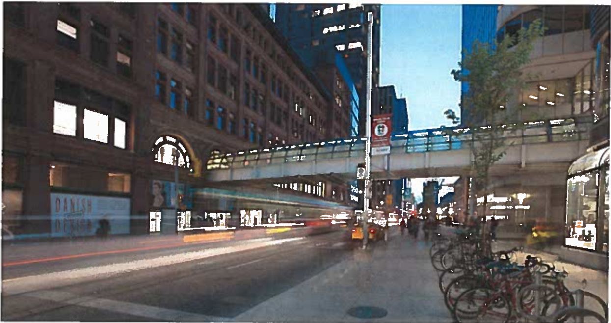
Photographs of existing Toronto Eaton's Centre Bridge
