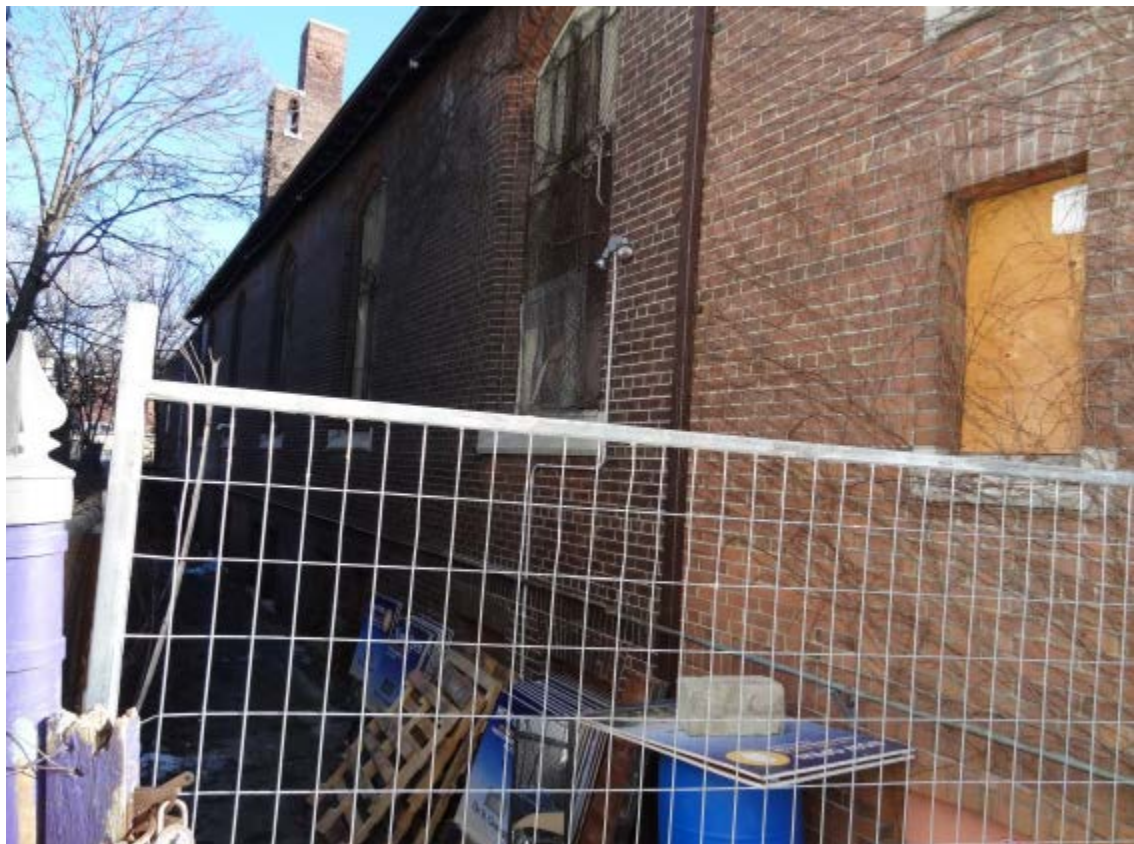
North Elevation – 175 Jones Avenue
