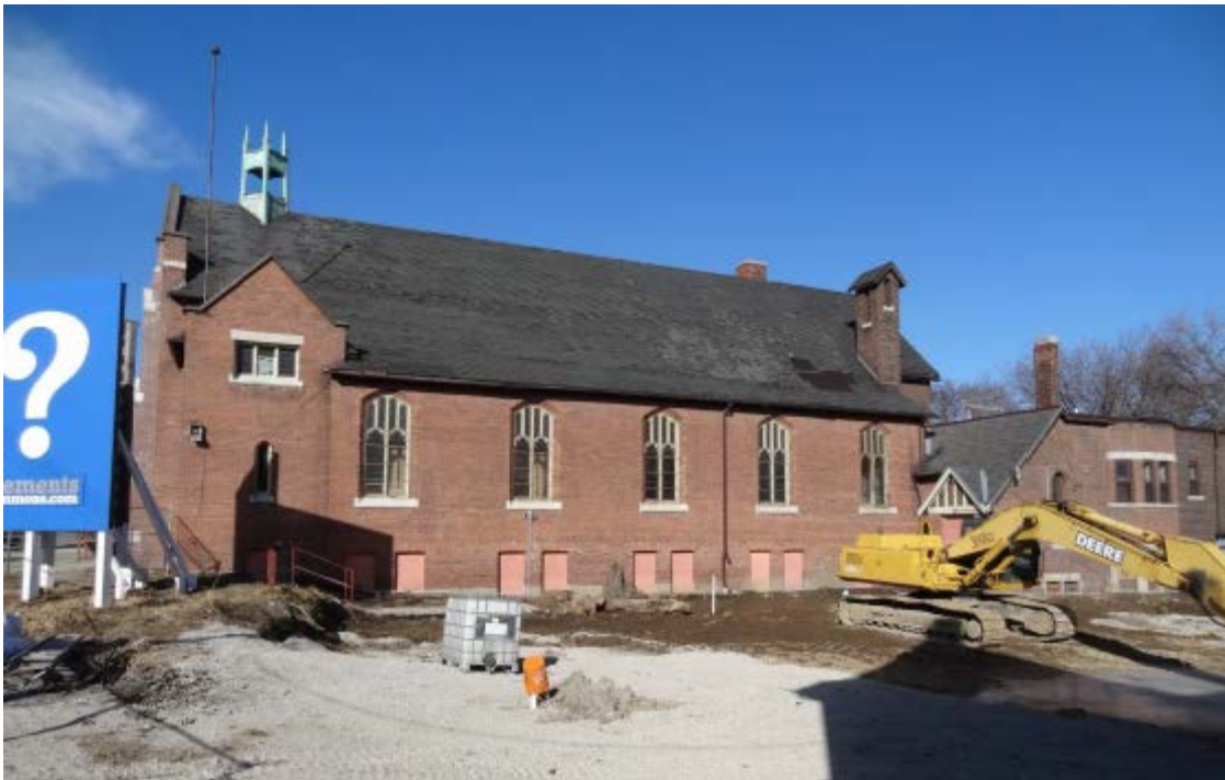
South Elevation – 175 Jones Avenue (Photo: AREA – July 31, 2015 HIA)
