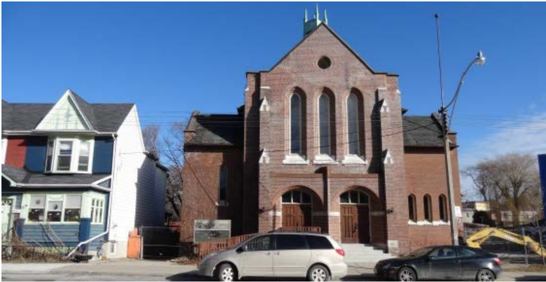
West Elevation – 175 Jones Avenue (Photo: AREA – July 31, 2015 HIA)
