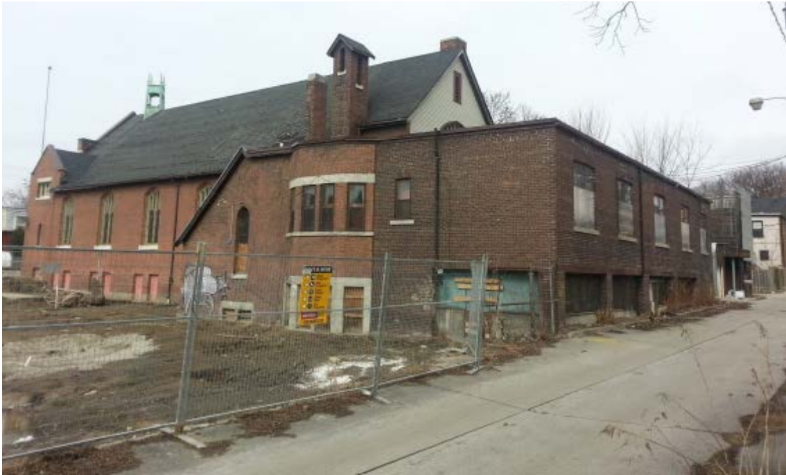
Southeast Corner – 175 Jones Avenue (Photo: AREA – July 31, 2015 HIA)
