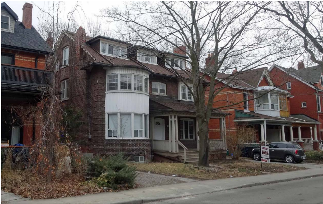
13. Current Photographs, 201 Crawford Street, February 2016 : showing the principal west elevation with the north (left) and south (right) elevations (above), and the context of the John Harkins House on the east side of Crawford Street (below) (Heritage Preservation Services, February 2016).
