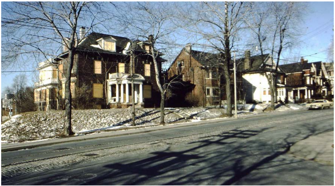
12. Archival Photograph, Broadview Avenue, north of Montcrest Boulevard, 1976 : showing the David Wagstaff House (third from the left) as part of the enclave of early 20 th century residential buildings in this block (Toronto Historical Board).
