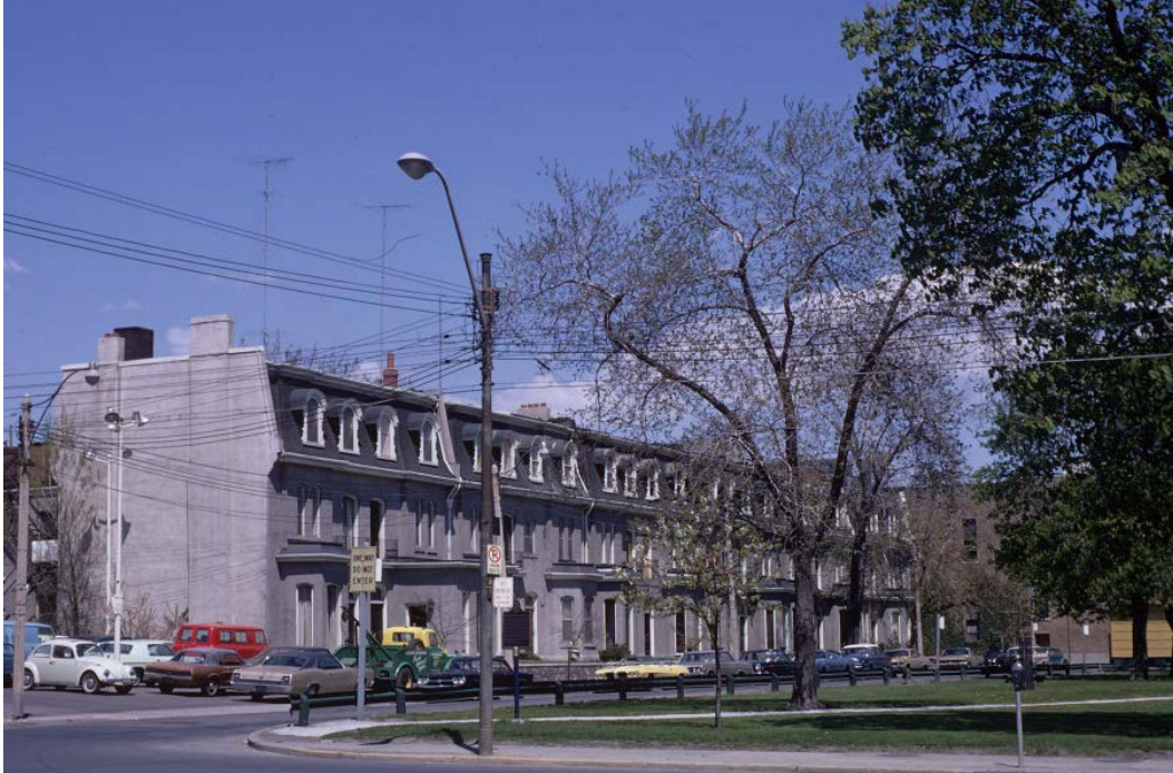
19. Archival Photograph, 5-16 Clarence Square, 1971 : the surviving section of the row houses (terrace) is shown overlooking the north end of Clarence Square. The houses date to the late 1870s and are recognized on the City of Toronto's Heritage Register (City of Toronto Archives, Fonds 1526, Item 91).
