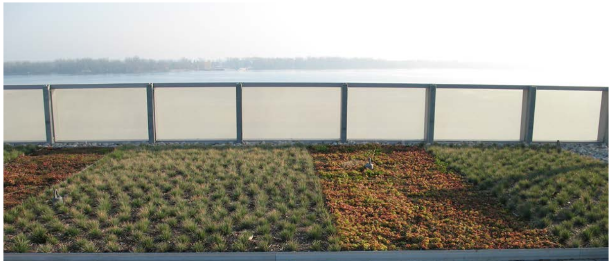
Figure 7.16 Green Roof, East Bayfront
