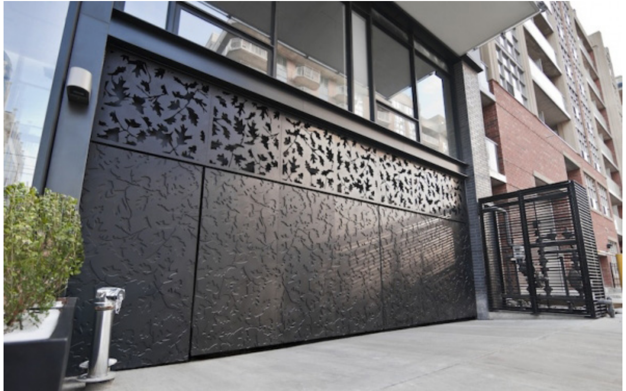
Figure 5.36 Parking and loading entrance
