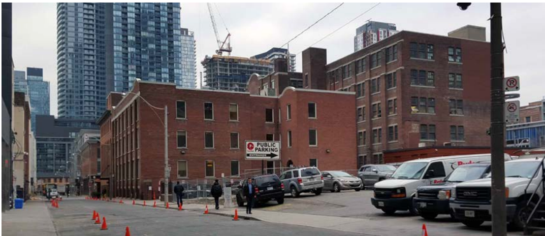
17. Current Photographs, 19 Duncan Street, 2016 : showing the west elevation on Duncan Street and part of the south elevation with the painted signage (above), and the view of the east elevation and part of the rear (south) elevation from Pearl Street (below) (Heritage Preservation Services).
