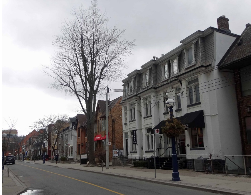
16. Current Photograph, Scollard Street, west of Bay Street, 2016: showing the heritage buildings that are part of the Yorkville-Hazelton Heritage Conservation District (2002), including the semi-detached houses at 72-76 Scollard (right) that were previously listed on the City Toronto Inventory of Heritage Properties (now known as the Heritage Register) in 1976 (Heritage Preservation Services).
