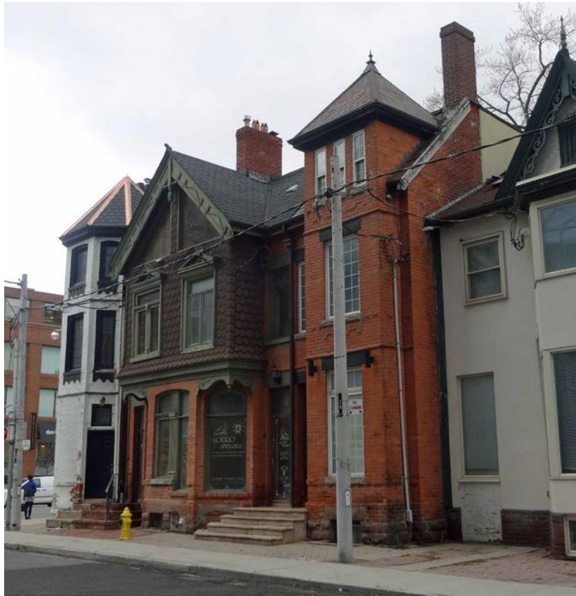
18. Current Photographs, 54A, 56 and 58 Scollard Street and 1315 Bay Street, April 2016 : showing the principal (south) elevations of the row houses (above) and the east (side) elevation of the unit at 54A Scollard (below) (Heritage Preservation Services).
