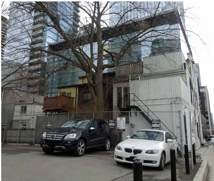
20. Current Photographs, 54A, 56 and 58 Scollard Street and 1315 Bay Street, April 2016 : showing the rear (left) and west (right) elevations of the row houses (above) and the rear elevations and addition from Bay Street (below, right) (Heritage Preservation Services).
