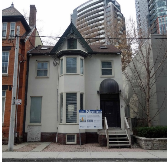
Principal (south) elevation, 54 Scollard Street (Heritage Preservation Services, 2016)
