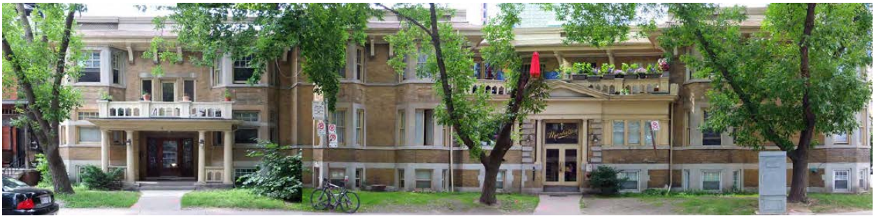
Manhattan Apartments, Charles Street East Elevation Phil Goldsmith Architect
