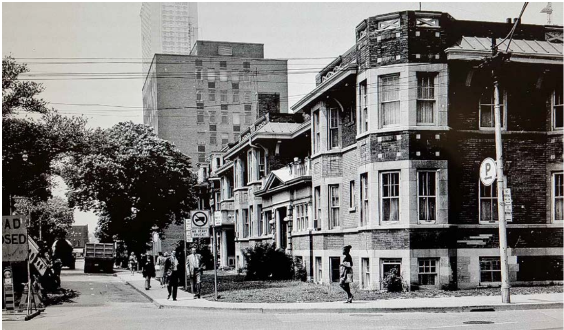
12. Archival Photographs, 628 Church Street, 1973 : contextual views looking north on Church Street (above) and west along Charles Street East toward Yonge Street (below) and showing the Manhattan Apartments at the northwest corner of the intersection (City of Toronto Archives, Fonds 2043, File 53).
