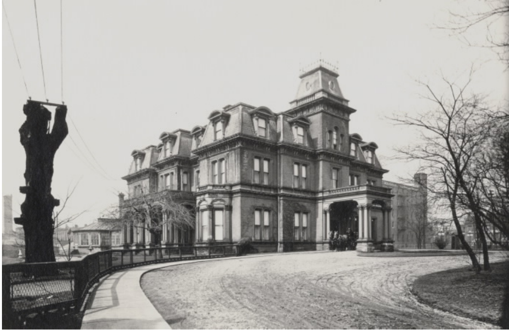
8. Archival Photograph, Government House, 1912 : documented prior to its demolition, the official residence of Ontario's Lieutenant-Governor at King and Simcoe streets with its Second Empire styling inspired residential architecture in the city (Toronto Public Library, Item 1792)
