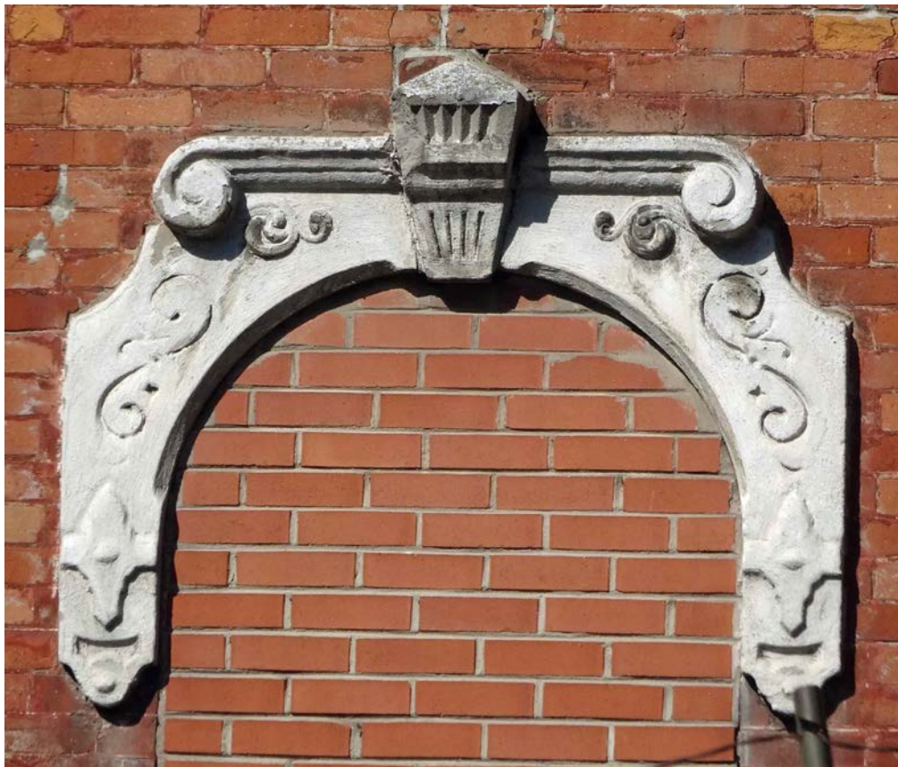
16. Current Photographs, 212 Dundas Street East, 2016 : view of George Street and the west elevations of the Henry Tasker House (above), and the stone detailing on one of the window openings on the east elevation (below) (Heritage Preservation Services).
