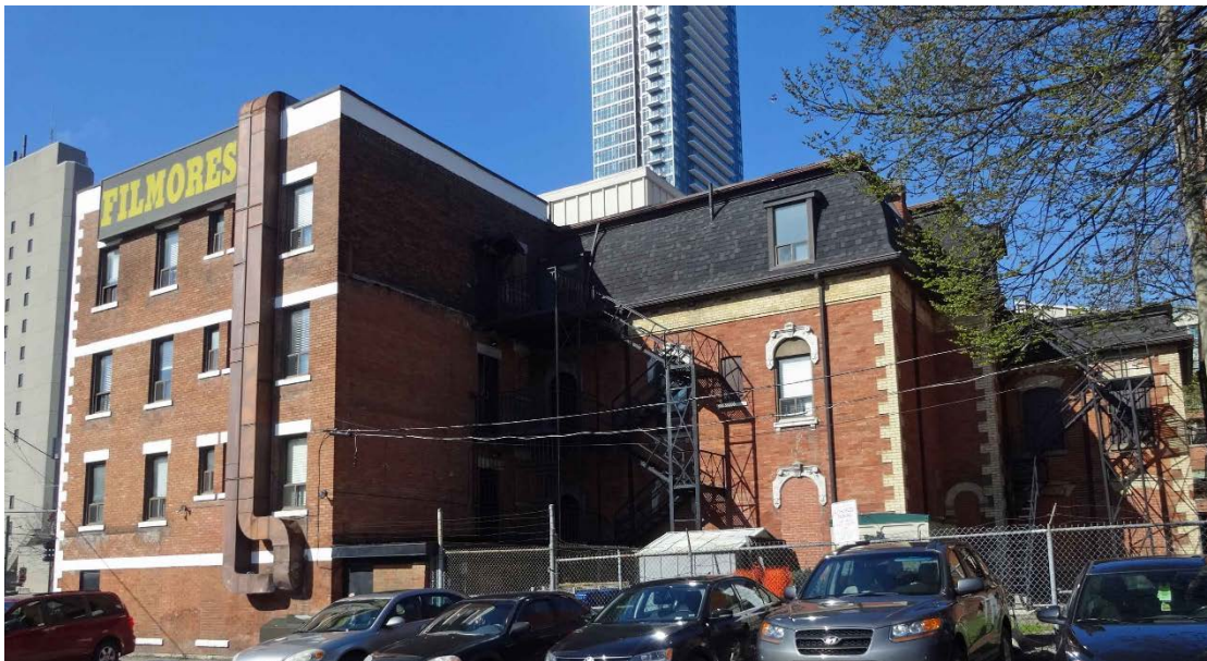
15. Current Photographs, 212 Dundas Street East, 2016 : showing the west elevations of the Wilton Court Hotel and the Henry Tasker House on George Street (above), and the east elevation and part of the rear (north) wall of the hotel where it adjoins the house and wing (below) (Heritage Preservation Services).
