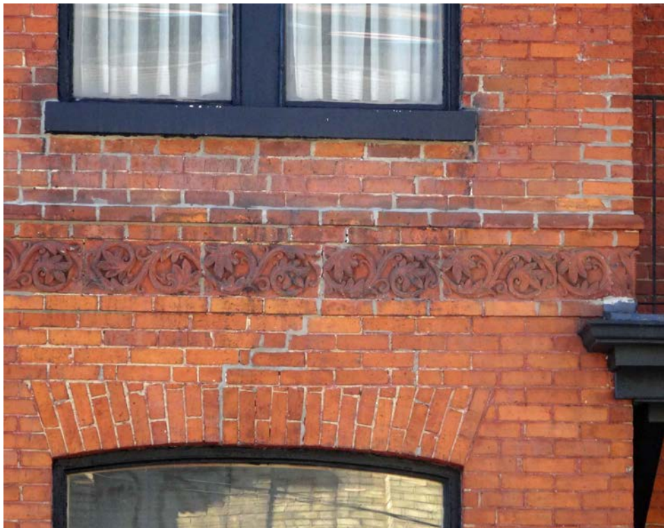
12. Current Photograph, 201 and 203 Gerrard Street East, 2016 : showing the rear (south) walls (above), and the detailing on the principal (north) elevations with the decorative terra cotta (below) (Heritage Preservation Services, 2016).
