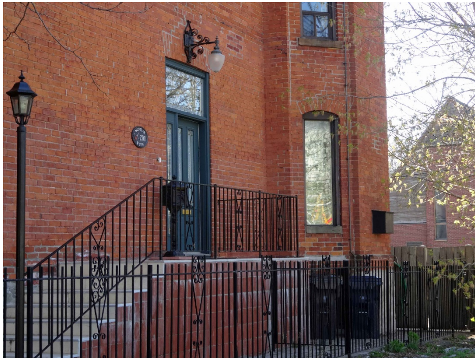
11. Current Photographs, 201 and 203 Gerrard Street East, 2016 : showing the west elevation of 201 Gerrard (above) and the entrance on this wall (below) (Heritage Preservation Services).
