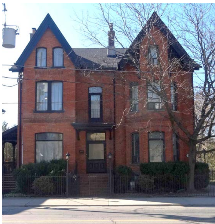
Cecilia Lloyd/Harry Rosser Houses: principal (north) elevations (Heritage Preservation Services, 2016)
