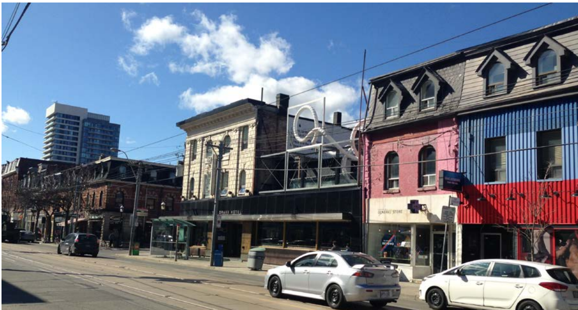
Showing the principal (south) elevations of 1144 and 1142 Queen Street West (top photo) and, looking west, beyond the Drake Hotel, the context of primarily late 19 th century, two-and-a-half to three-and-a-half storey, brick-clad, mansard-roofed, commercial blocks (bottom) ( Heritage Preservation Services, 2016 )
