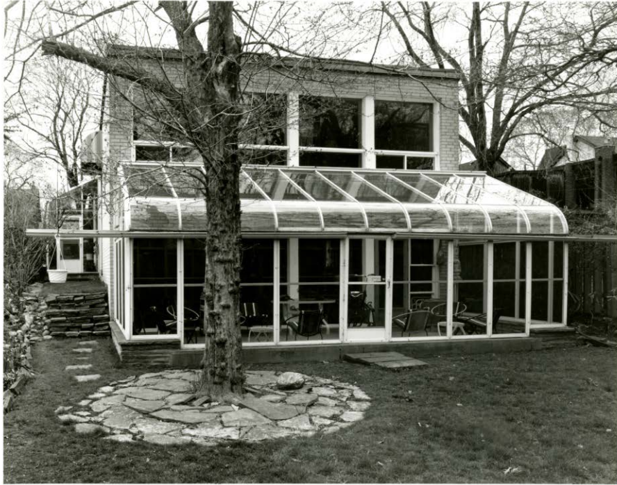
York Wilson House, Rear (South) Elevation (1997)
