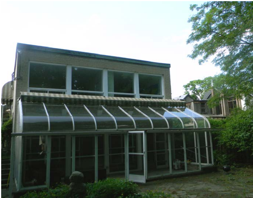
York Wilson House, Rear (South) Elevation, Heritage Preservation Services (2016)
