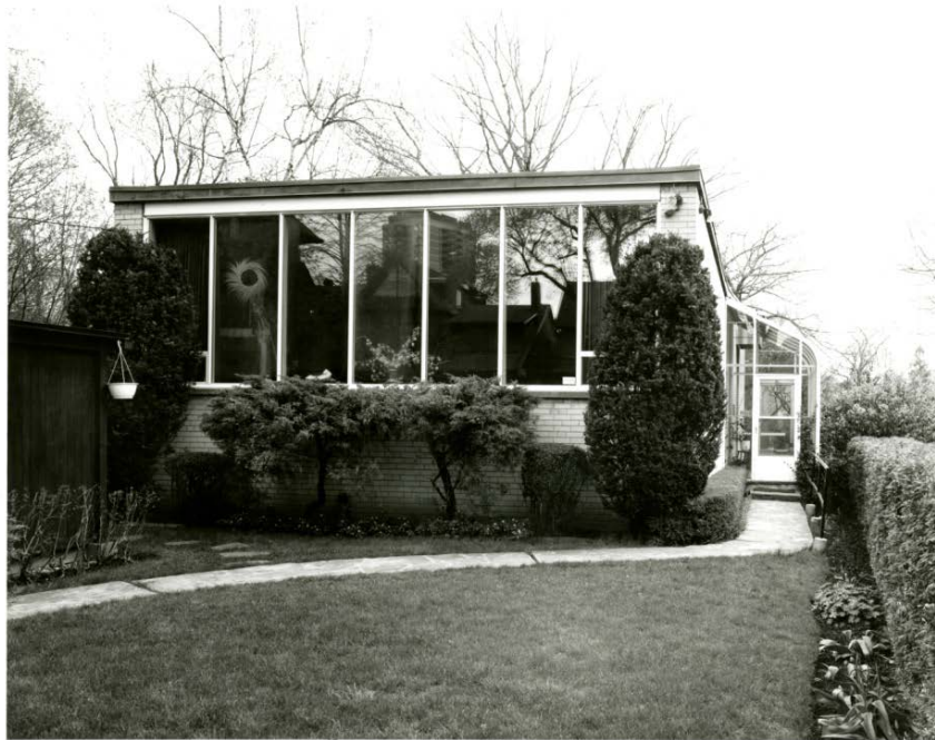
York Wilson House, Front (North) Elevation (1997)
