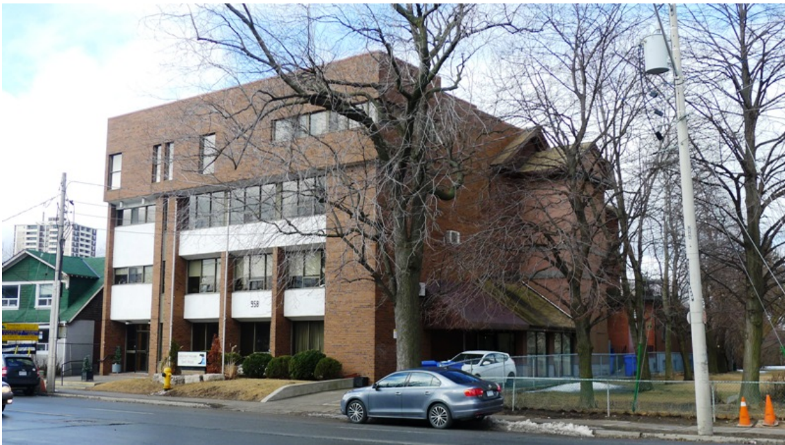
21. Chester School with Estonian House Additions, 1975 and 1995 : showing the addition from the north east. Note the original gable roof of the school. The single storey addition with the gable roofed addition in front of the school was completed in 1995 with the installation of an elevator (HPS)
