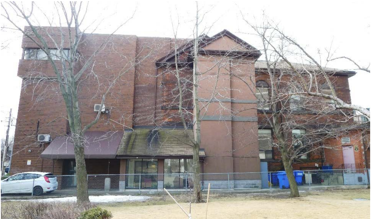
31. North Elevation: showing the one storey entry addition with the new tower for the elevator. The material of the addition, EIFS, is distinct from the brick but in a complementary colour. The decorative coursing bands further integrate the new with the old while maintaining a distinction between the two. The 1975 addition can be seen at the far left and the original school at the left and right of the tower. (HPS)
