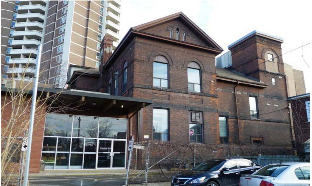
12. South Elevation : showing the tower and projecting bay with the triple arched windows in the gable end and the tower. Note also the stone and brick string courses. The 1962-3 addition and its entry is shown at the left of the photo (HPS)
