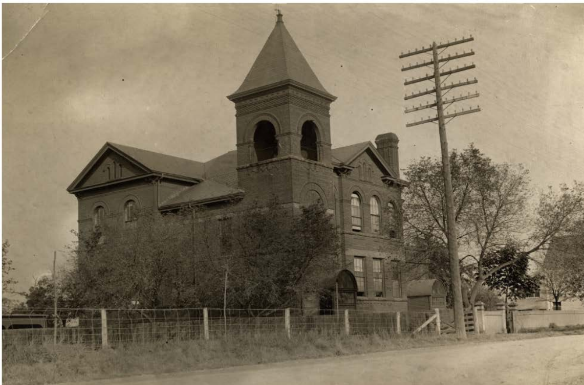
10. Chester Public School, Broadview Avenue, west side between Chester Hill Road and Helliwell St., 1905 : showing the south and east elevations. (TEC409, Baldwin Collection B13-16, Toronto Public Library)
