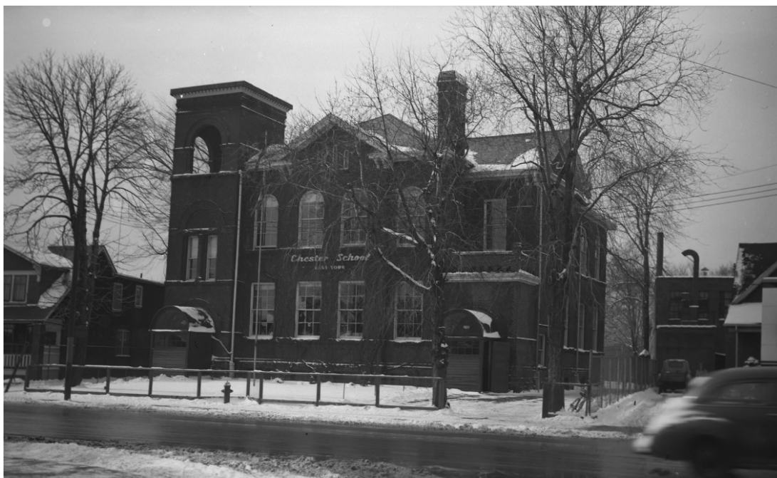
11. Chester Public School, Broadview Avenue, west side, between Chester Hill Road and Helliwell Street, 1953 : showing the east and north elevations after the removal of the pyramidal tower roof (James Victor Salmon (1911-58), Baldwin Room, S1-1236, TPL)
