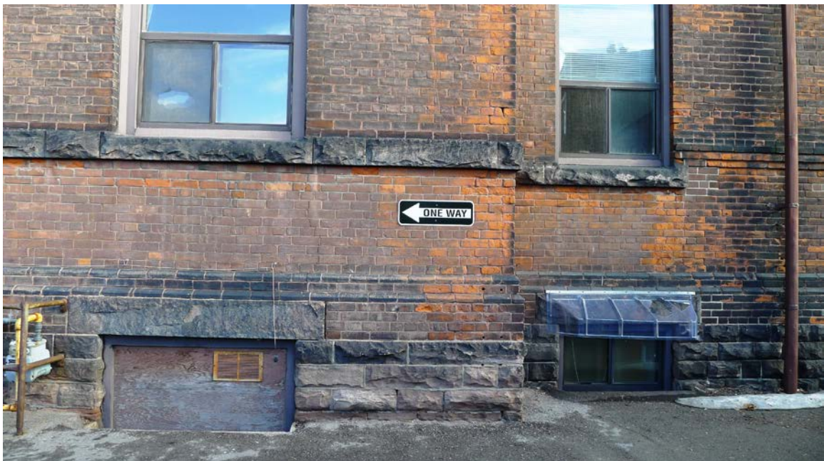
13. South Elevation, detail : showing the basement and first floor walls with stone rusticated stone foundation, lintels, sills and string courses and the decorative brick string courses (HPS)
