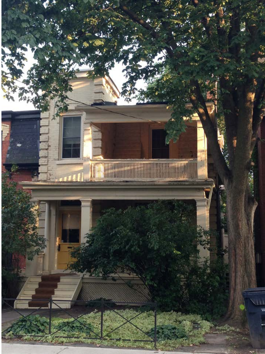
33 Sussex Avenue, north (principal) elevation ( HPS )
