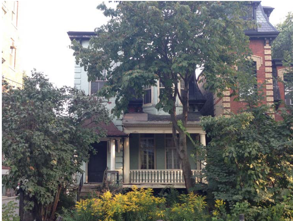
29 Sussex Avenue, north (principal) elevation ( HPS, 2016 )
