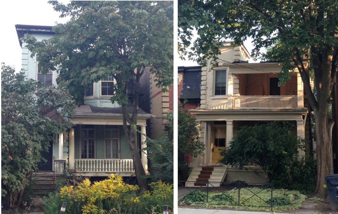
29 Sussex Avenue (left) and 33 Sussex Avenue (right) (HPS, 2016)
