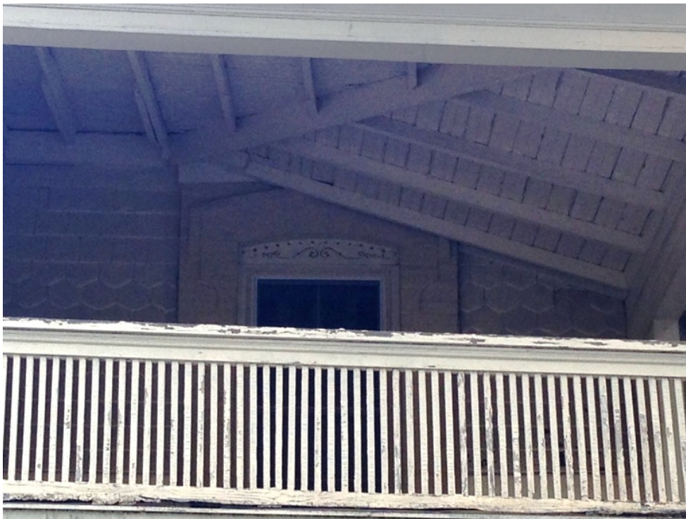
14. 33 Sussex Avenue : showing the second floor, underneath the verandah roof, with the original slate roof with its plain and fish-scale slates and the original window with the brick and wood details (HPS 2016)
