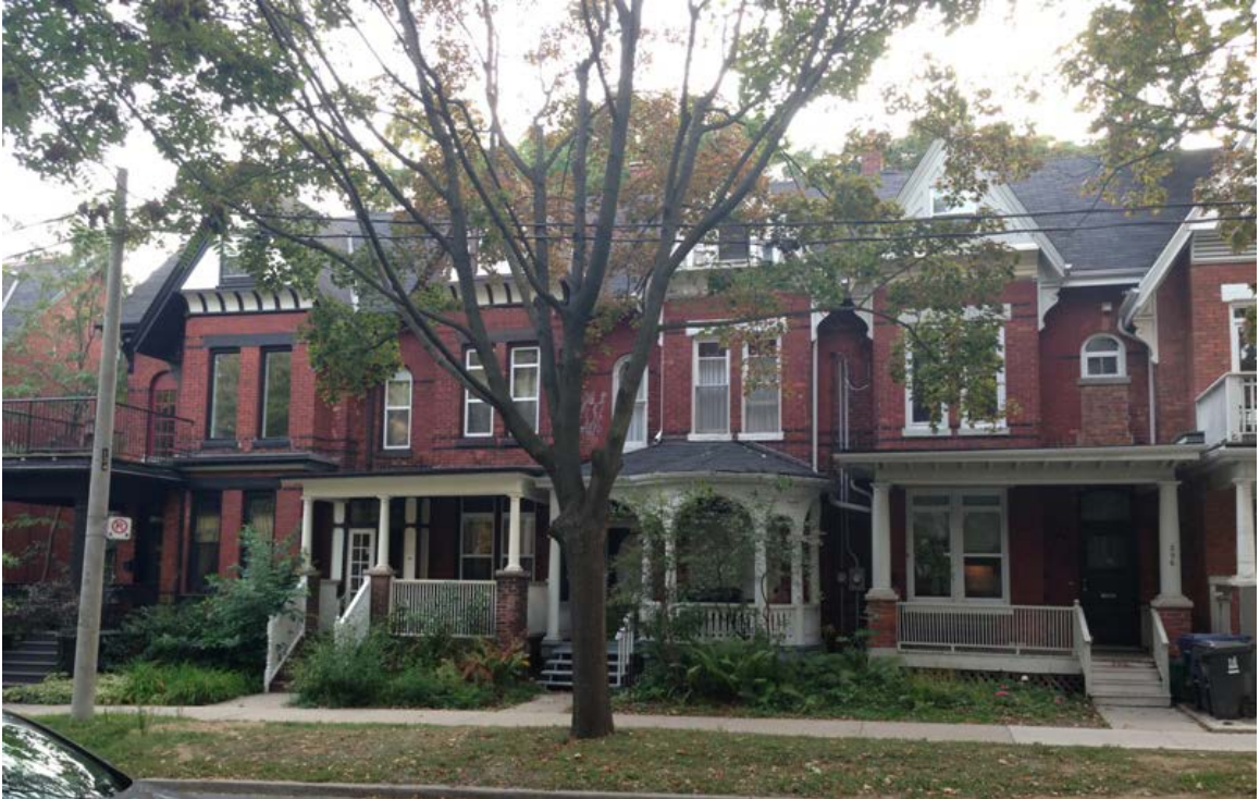
28. Huron Street, west side, north of Sussex Avenue (HPS, 2016)
