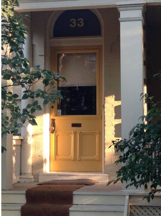
17. 33 Sussex Avenue : showing the door with its panelling and hardware and the fanlight (HPS, 2016)
