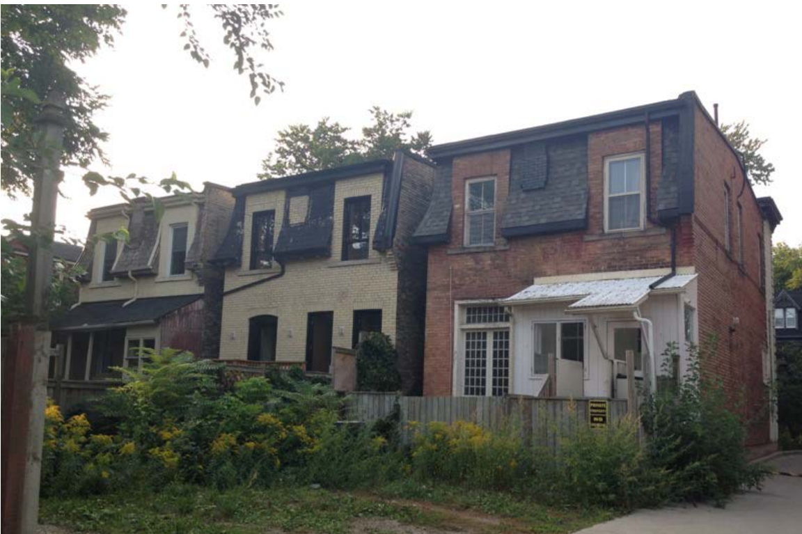
20. Rear (South) Elevations at 33, 31 and 29 Sussex Avenue ; showing the parapet walls on the east elevations instead of mansard roofs and the buff brick cladding at 33 and 31 Sussex and, at 29 Sussex, the red wash applied to the rear and side walls (HPS, 2016)
