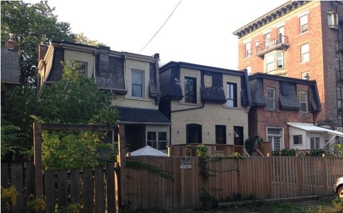
19. Rear (South) Elevations at 33, 31 and 29 Sussex Avenue ; showing the mansard roofs on the west and south elevations and the parapet wall on the east. (HPS, 2016)
