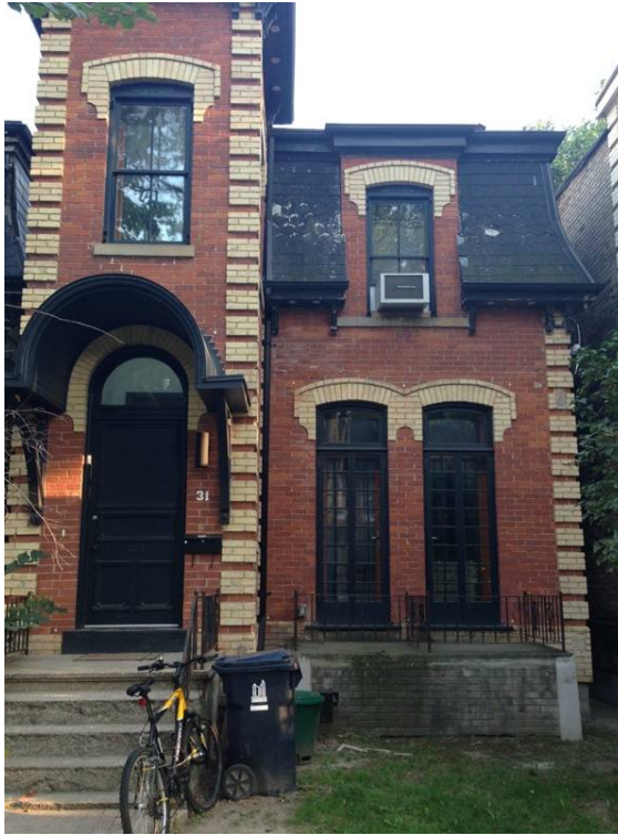
13. 31 Sussex Avenue : showing the mansard roof, the paired French doors, the decorative yellow brick trim with the yellow brick chaine at the corners. (HPS 2016)
