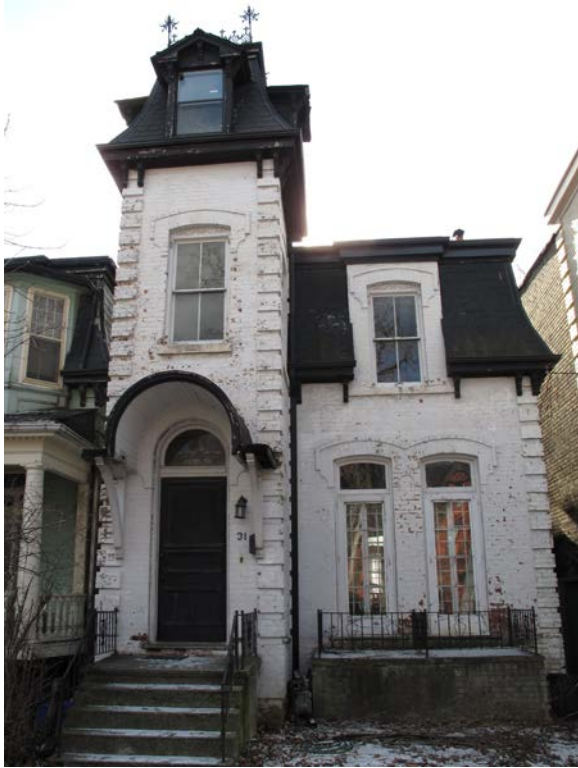
7. 31 Sussex Avenue, 2013 : showing the house prior to the restoration. (ERA Architects, Inc.)
