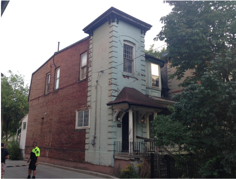
21. 29 and 31 Sussex Avenue : showing the north (front) and east(side) elevations of 29 Sussex Avenue. Note the buff brick evident on the side of the tower at 31 Sussex Avenue.
