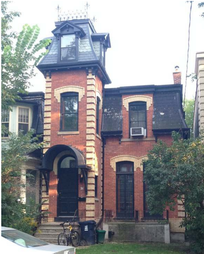
8. 31 Sussex Avenue : showing the house after restoration (HPS, 2016)
