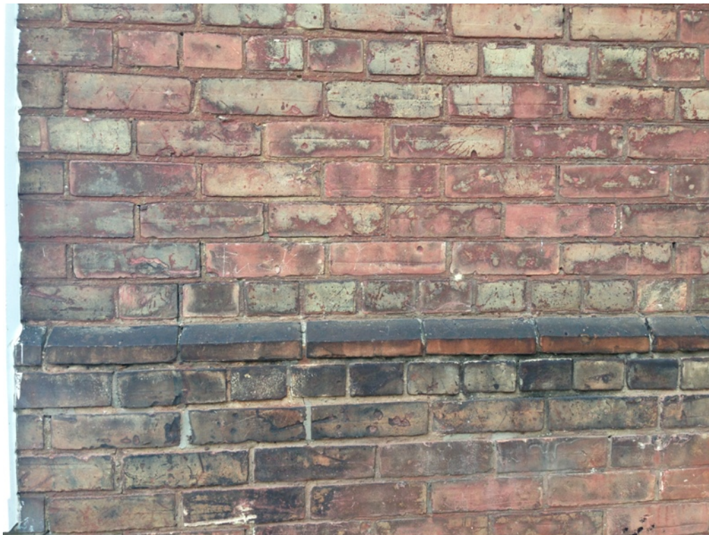
22. 29 Sussex Avenue, East (Side) Elevation : showing the remnants of the red wash applied over the buff brick (HPS 2016)
