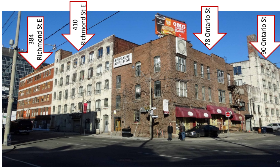
Photograph of the northwest corner of Ontario Street (right) and Richmond Street East (left), showing the industrial buildings adjoining the intersection, which are individually identified by the arrows (Heritage Preservation Services, 2016).
