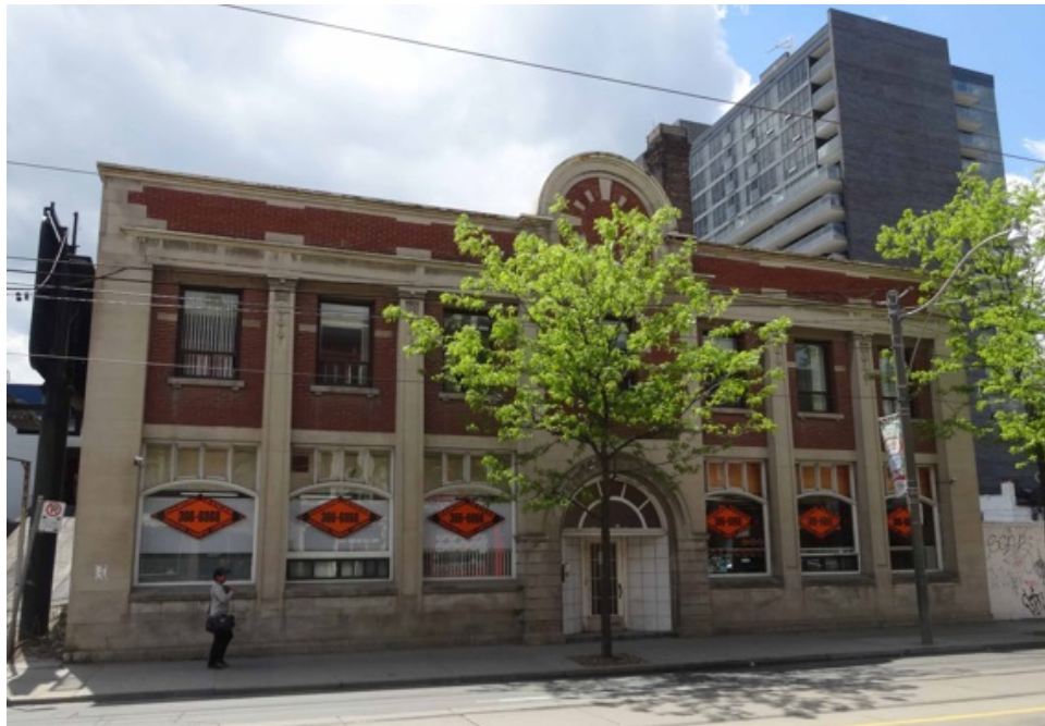
Photograph of the S. Price and Sons Dairy Building at 245 Queen Street East, showing the principal (north) elevation (Heritage Preservation Services, 2016).
