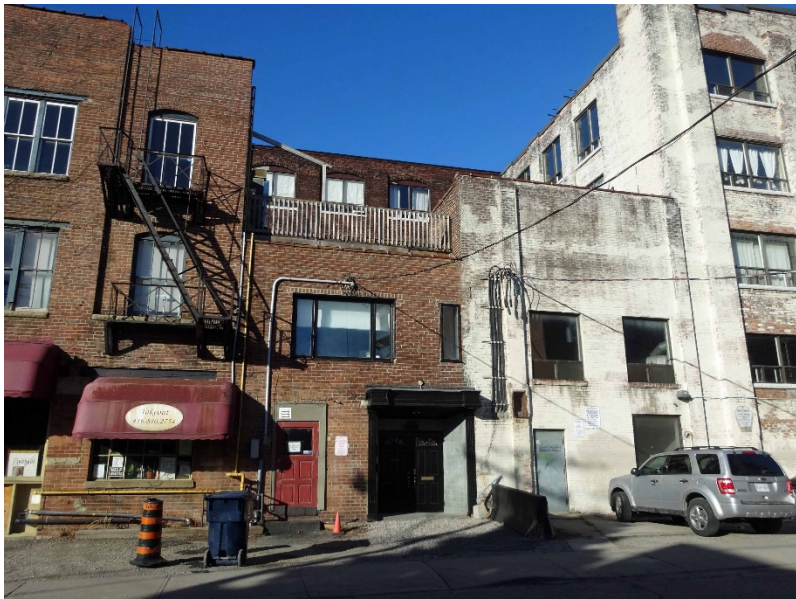
14. Current Photographs, Newell Building, 90 Ontario Street, 2016 : showing the north elevation of the Newell Building adjoining Brigden Place (above), and south elevation that is visible above the low-rise building at 88 Ontario Street (below right). While part of the Newell Company's complex, the latter building is not identified as a heritage attribute (Heritage Preservation Services, 2016).
