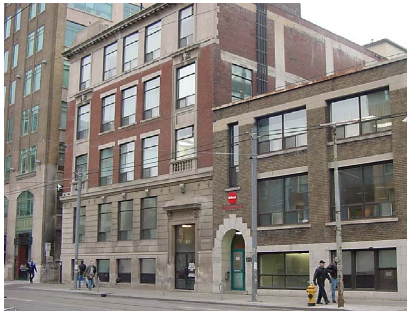
12. Photographs, Lever Brothers Building, 21 Don Roadway, 1920 (above), and Ellis Building, 384 Adelaide Street East, 2005 (below): showing two of the extant projects by William Sparling, architect for the building at present-day 384 Richmond Street East, both dating to the 1920s and with the exposed concrete grid with brick panels that he employed afterward on the Dominion Envelope Company Building (Toronto Public Library, LocHist-RD-015, and Heritage Preservation Services, 2005).
