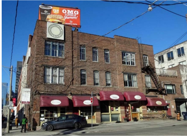
Above: principal (east) elevation of the Hamilton Brewing Association Building on Ontario Street; cover: east and south elevations on Ontario Street and Richmond Street East, respectively (Heritage Preservation Services, 2016)
