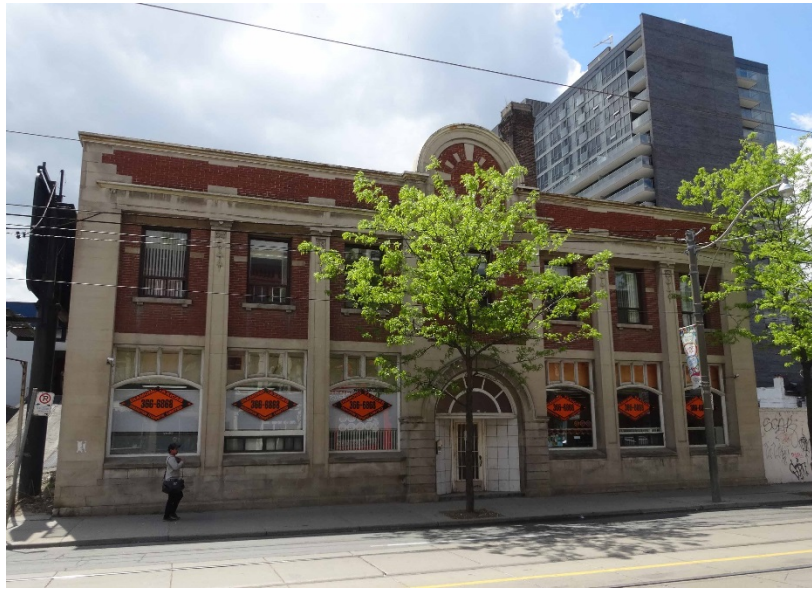
Above: principal (north) elevation of the S. Price and Sons Dairy Building at 245 Queen Street East; cover: north and east elevations (Heritage Preservation Services, 2016)
