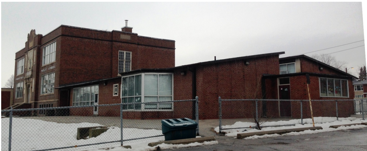
Vincent Massey Childcare Centre, showing the east addition (1956) (HPS, 2016)
