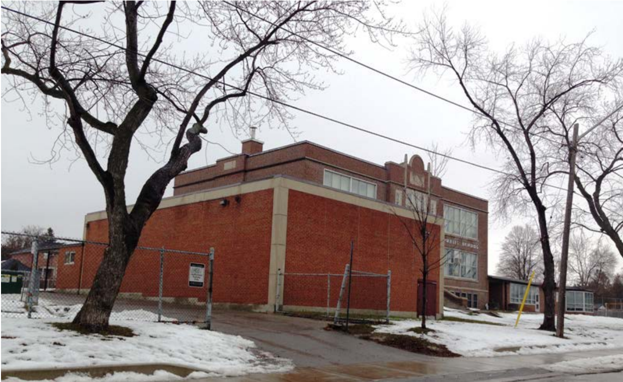
23. West addition: showing the principal (south) and side (west) elevations of the 1963-4 addition (HPS 2016)
