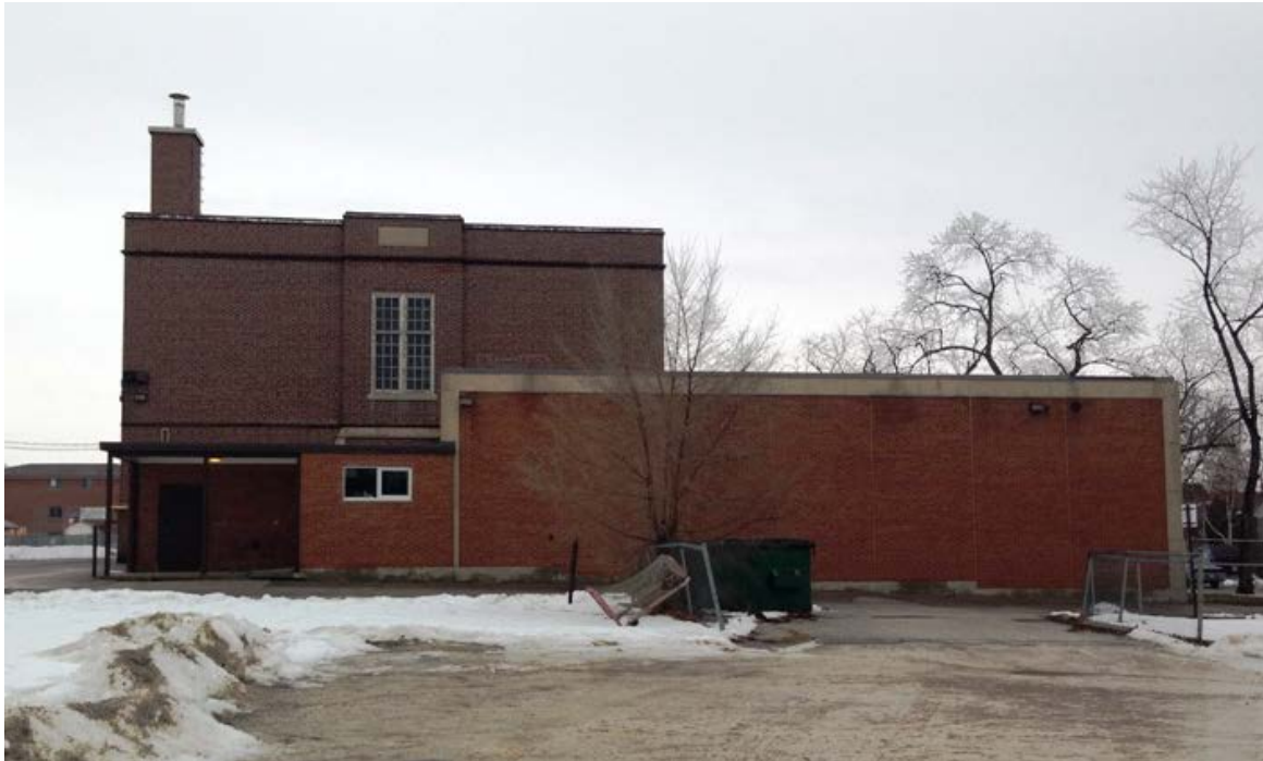
11. 68 Daisy Avenue: showing the side (west) elevation with the later 1963-4 addition (HPS, 2016)
