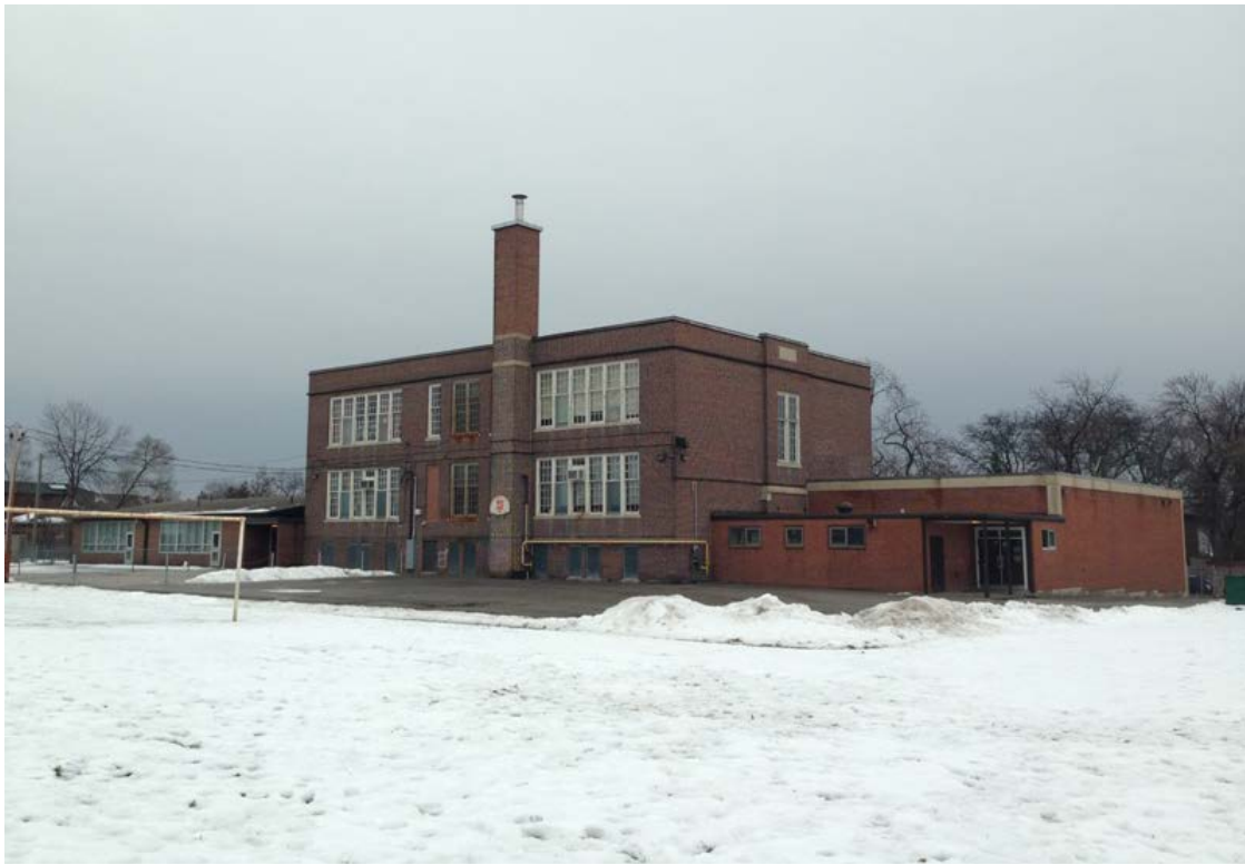
View from the north-west of the playground of the rear (north) elevations of the school and additions on the east and west sides (HPS, 2016)
