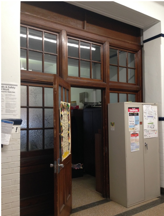
15. Second floor entry to offices showing the original wood details and glazing including the frosted glazing of the lower panels, the brick surface of the lower wall area, with a moulding and plaster above. (Above, left, HPS, 2017)
