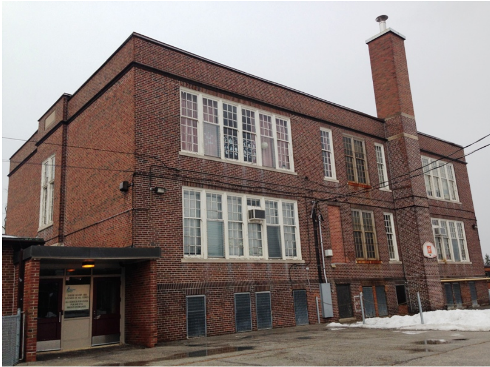
14. North (rear) elevation: showing the original wood double-hung sash windows with their nine-over-twelve sash. (HPS, 2016)
