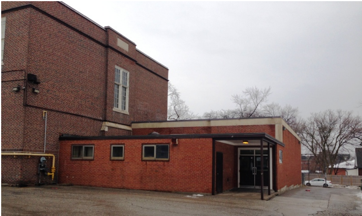
24. West Addition: showing the rear (north) elevation and entrance (HPS, 2016)
