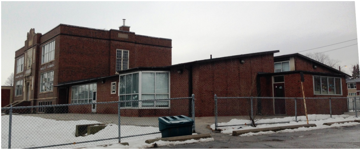
12. 68 Daisy Avenue: showing the side (east) elevation with the 1955-6 addition (HPS, 2016)
