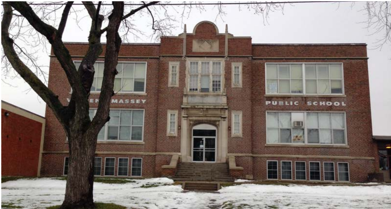
10. 68 Daisy Avenue, (1929): showing the principal (south) elevation (HPS, 2016)
