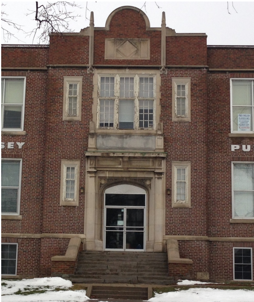
13. 68 Daisy Avenue, principal (south) elevation, central entry bay detail: showing the Tudor Revival elements combining Classical elements treated with a Collegiate Gothic style (HPS, 2016)
