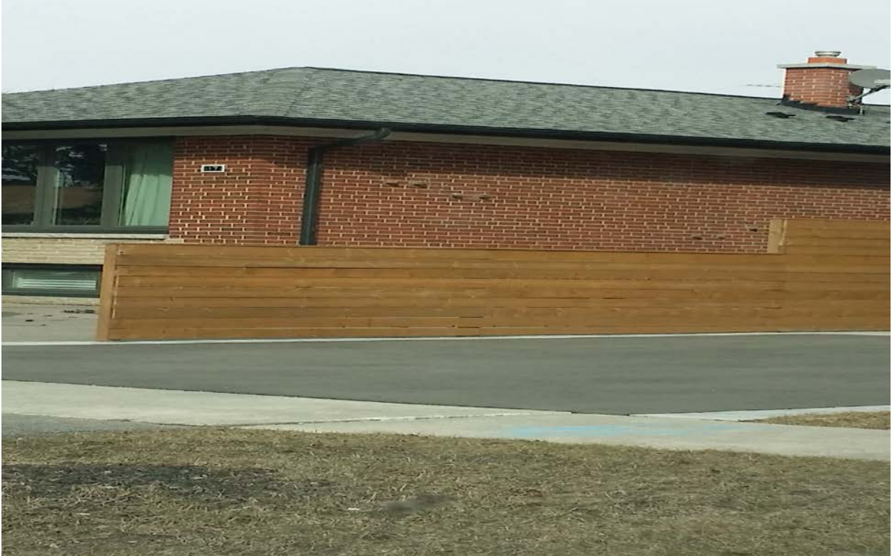
Attachment 3: Fence as seen facing North from 15 Stockbridge Avenue.
