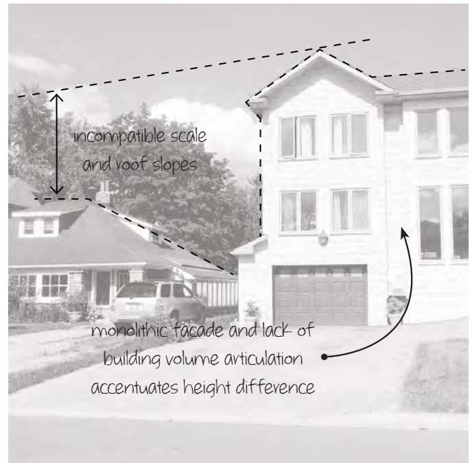
Figure 48 Incompatible building volumes accentuate height difference
