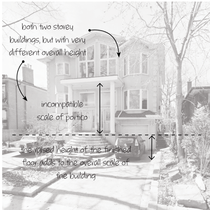
Figure 56 Front entry design emphasizes height discrepancy with adjacent buildings
