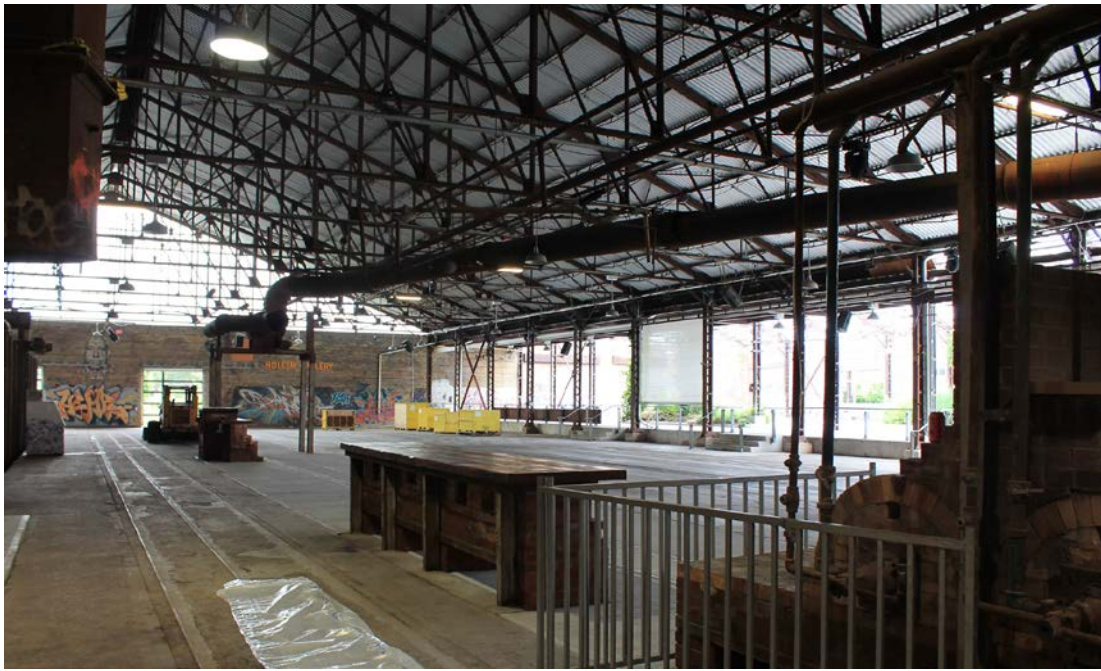
Interior of Building 16 looking south showing the open west wall (right,) proposed to be enclosed with glazing, and the network of interior railway tracks embedded in the floor (ERA Architects Inc.)
