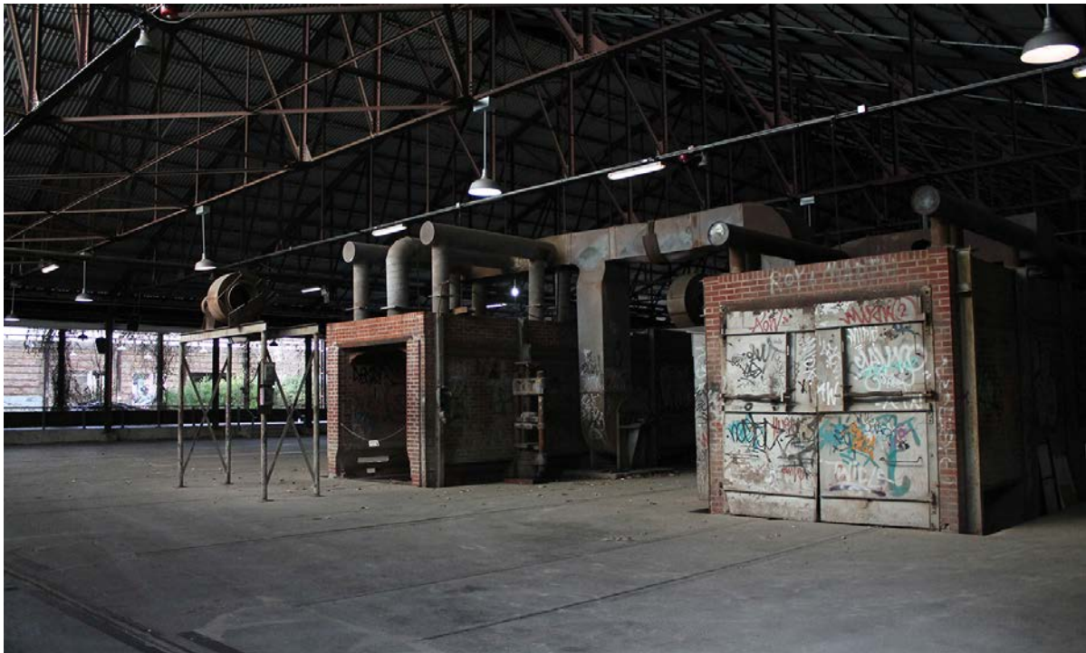
Interior of Building 16 showing the south ends of the firing kilns (ERA Architects Inc.)
