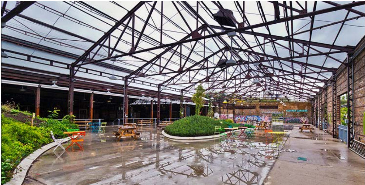
West Elevation of Building 16 as seen from within Building 15 (ERA Architects)
