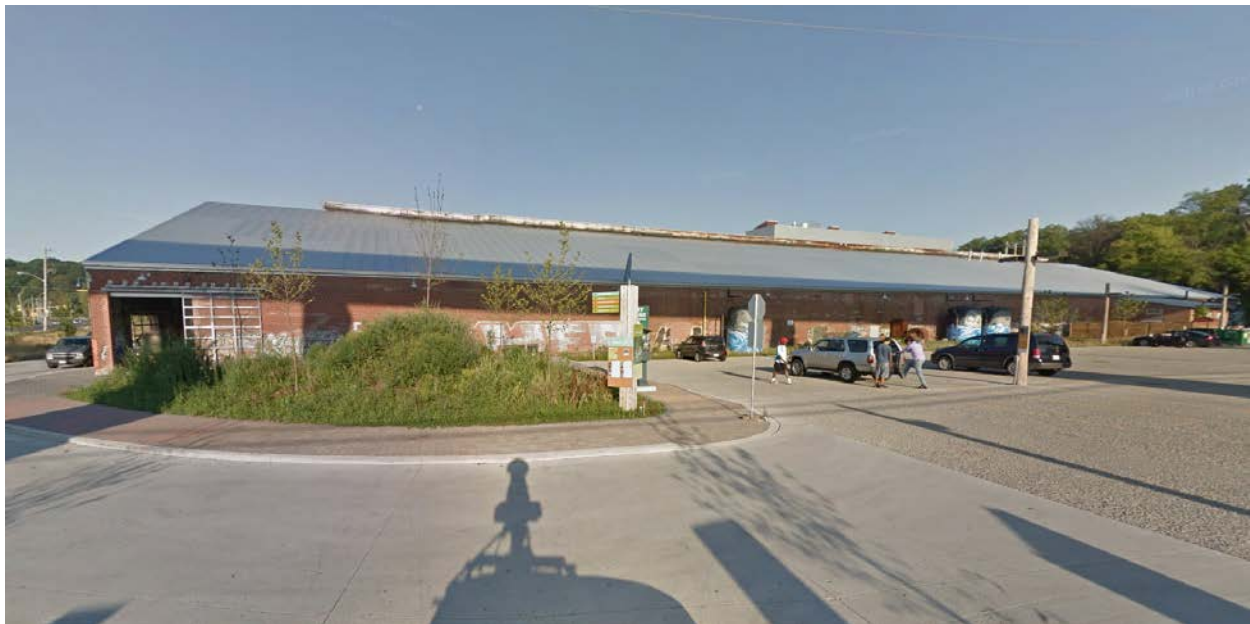
East Elevation of Building 16 (ERA Architects, Googlemaps, 2016)
