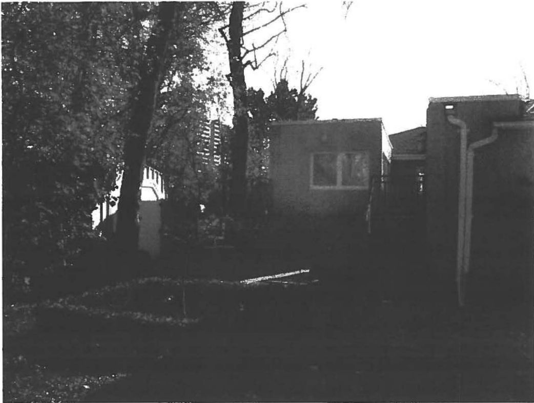
View of existing rear elevation, east side
