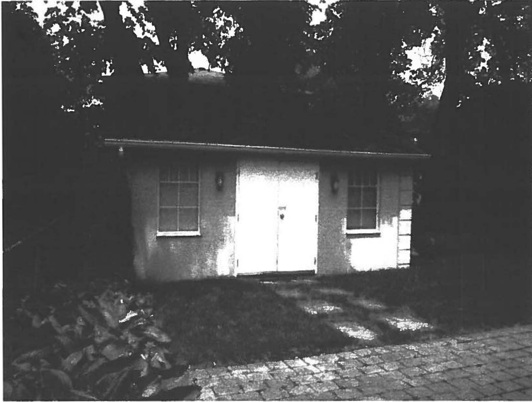
Existing Garden Storage Shed
