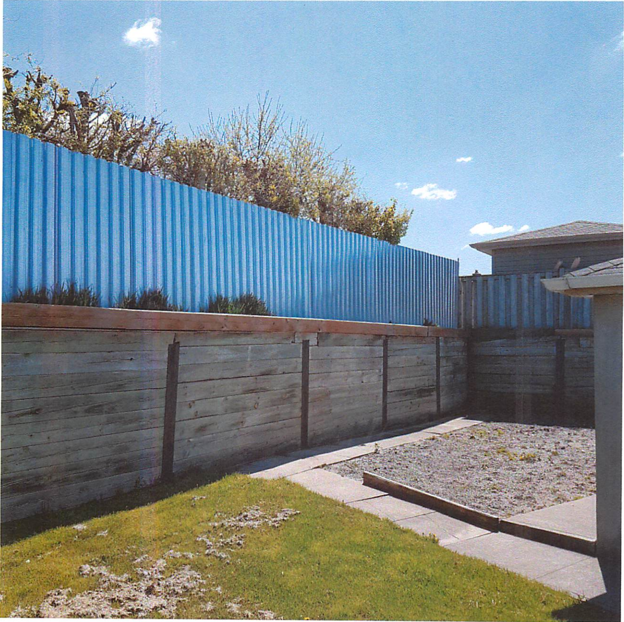
Attachment 2: Fence on West Side of Property
