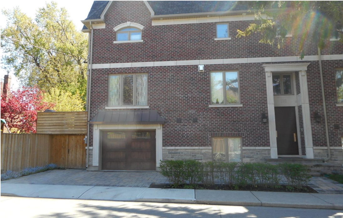
320 Brookdale Avenue (Elm Road flank) – May 17, 2016
