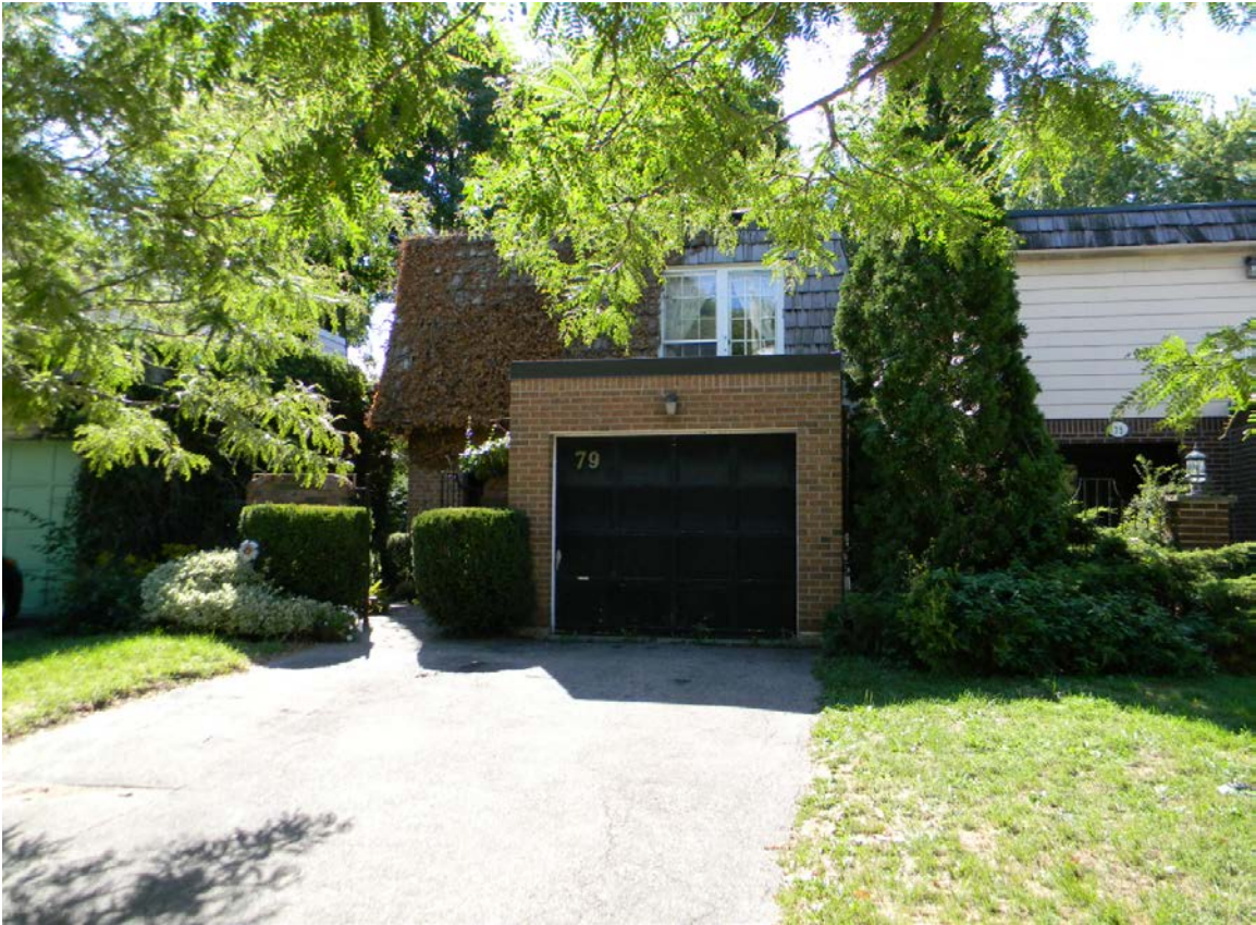
View of property looking south from Blythwood Road Heritage Preservation Services (2016)
