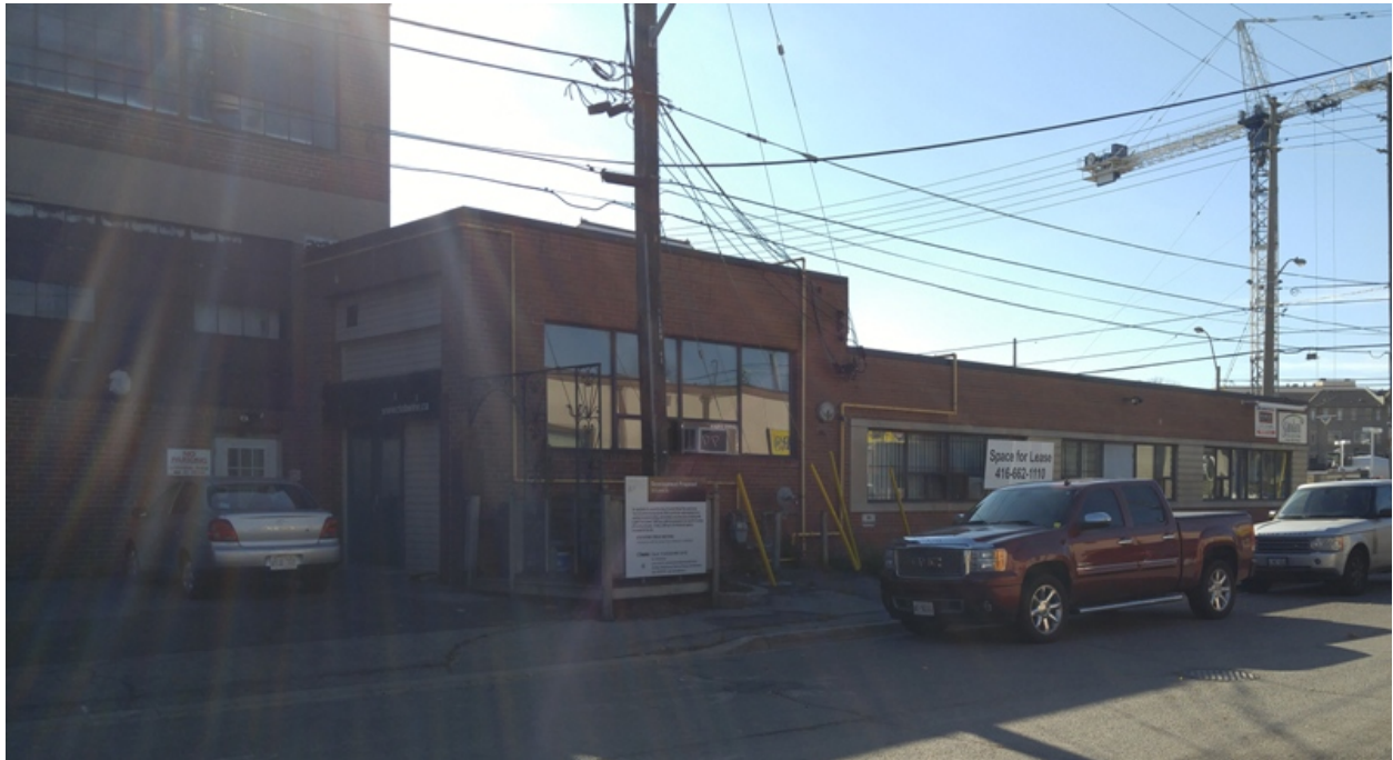
33 Laird Drive: showing the North Elevation (HPS 2016)
