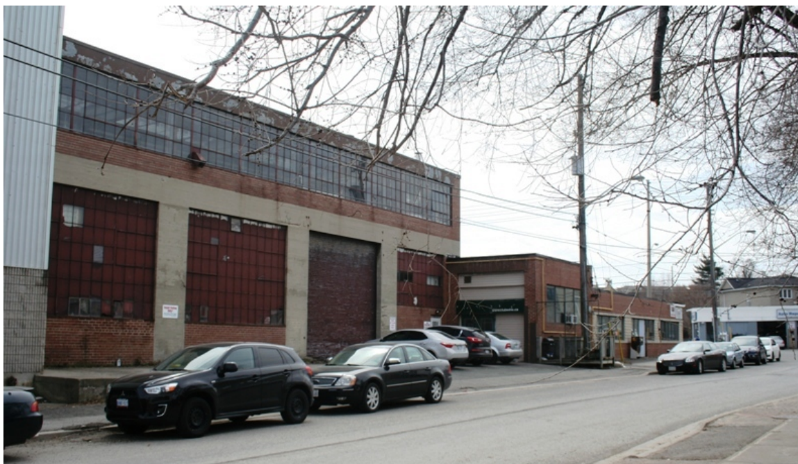
24. Sheridan Equipment Co. Ltd., north elevation: showing the two-story equipment repair workshop, the small loading bay office and, at the far right, the offices/stock rooms. (Heritage Preservation Services)
