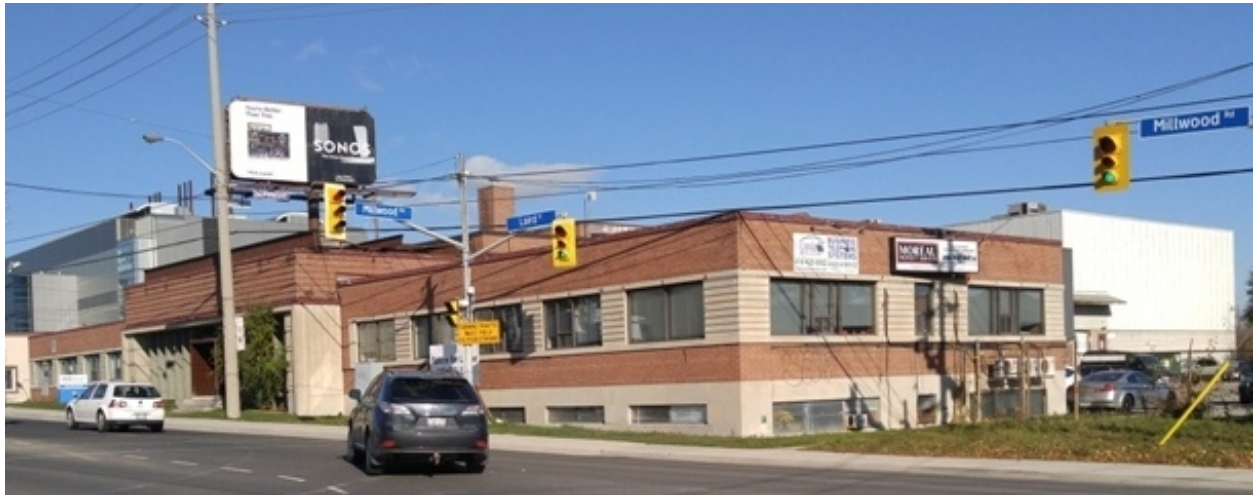
33 Laird Drive: showing the West and South Elevations (HPS 2016)
