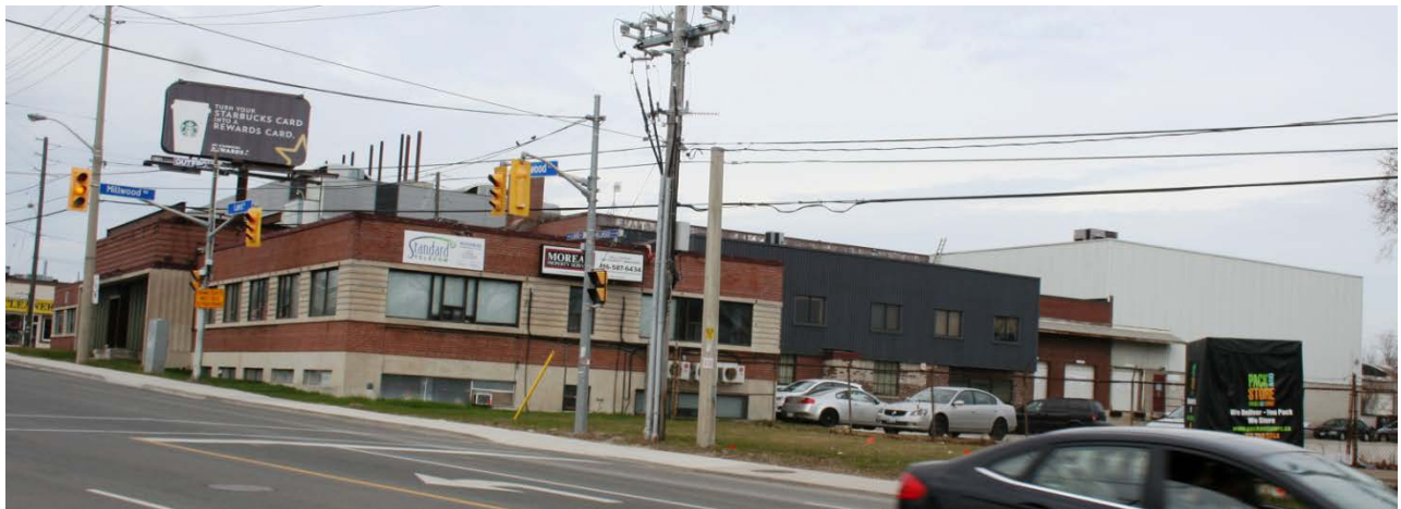
19. Sheridan Equipment Company Ltd., south-east elevations: showing the later extensions (clad in white metal) and the second storey addition (clad in black aluminum siding). (Heritage Preservation Services, 2015)
