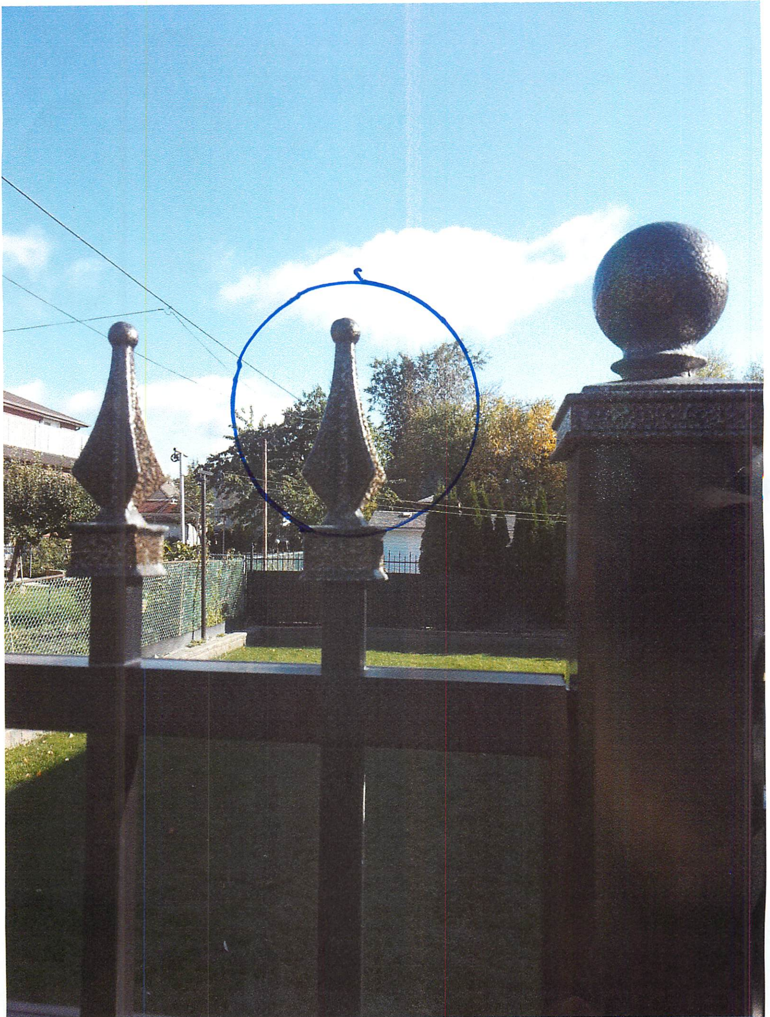
Attachment #6 - close up of wrought iron decorative tops
