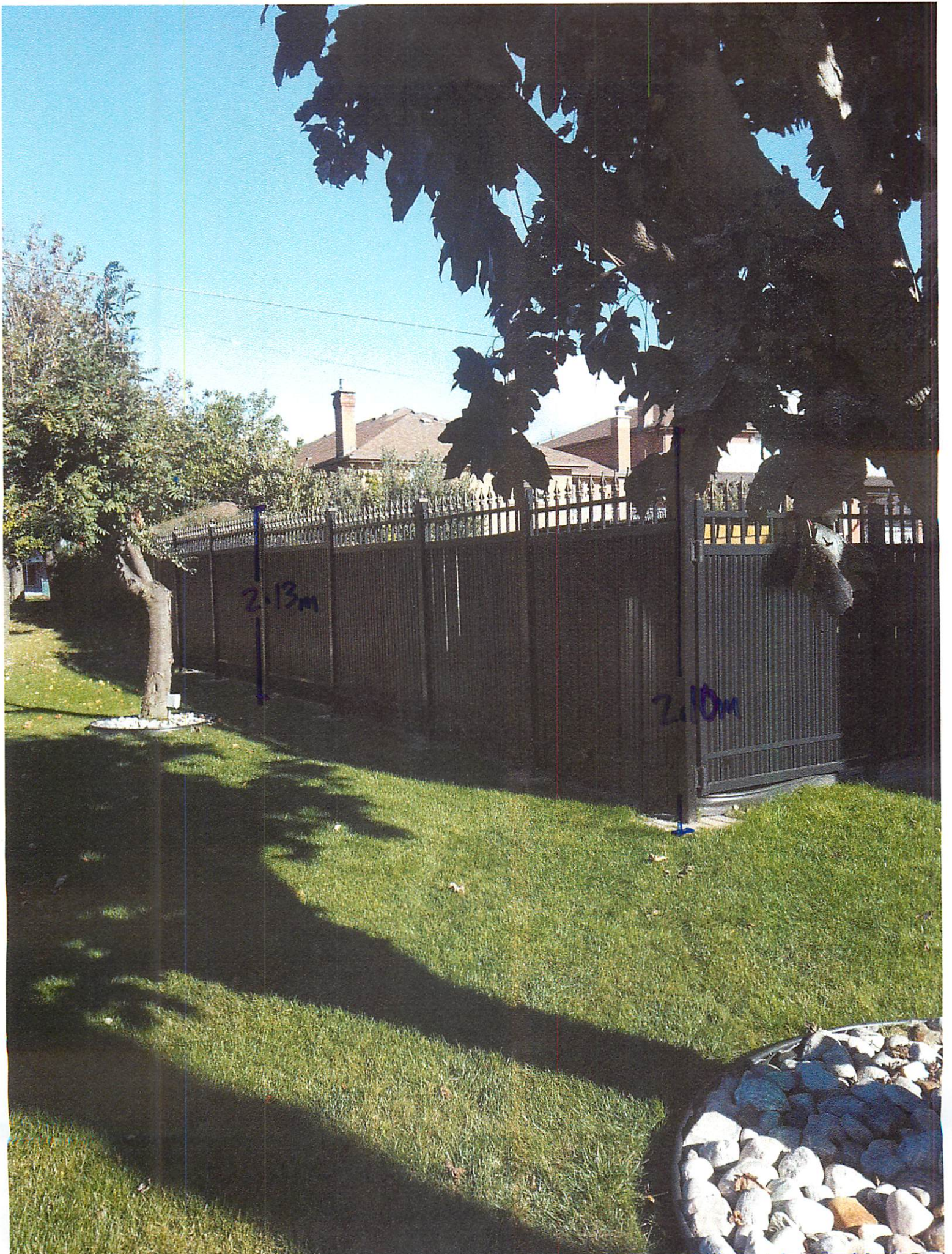
Attachment #4 - Section of fence @ west side of property
