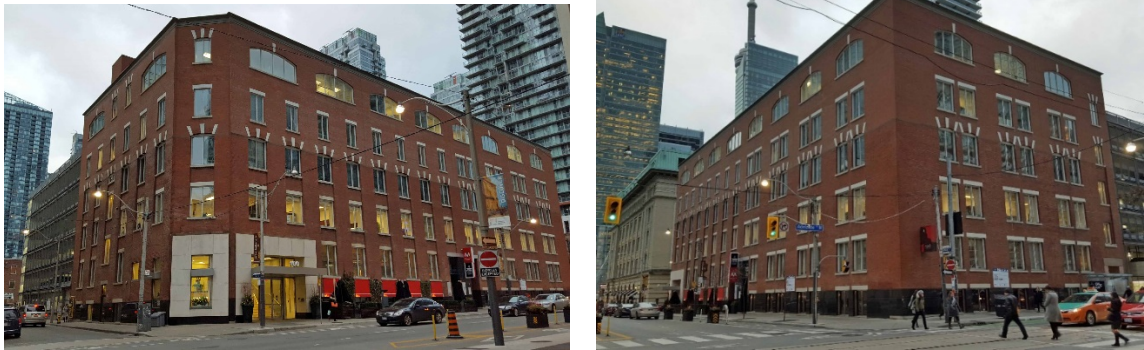
Above: south section (1904) adjoining Simcoe and Pearl streets (left), and north section (1905) adjoining Simcoe and Adelaide streets (right); cover: east elevation on Simcoe Street (Heritage Preservation Services, 2016)
