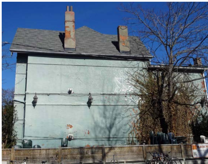
581 Markham Street: showing the south elevation at the north-east corner of Markham and Lennox Streets (HPS, 2015)
