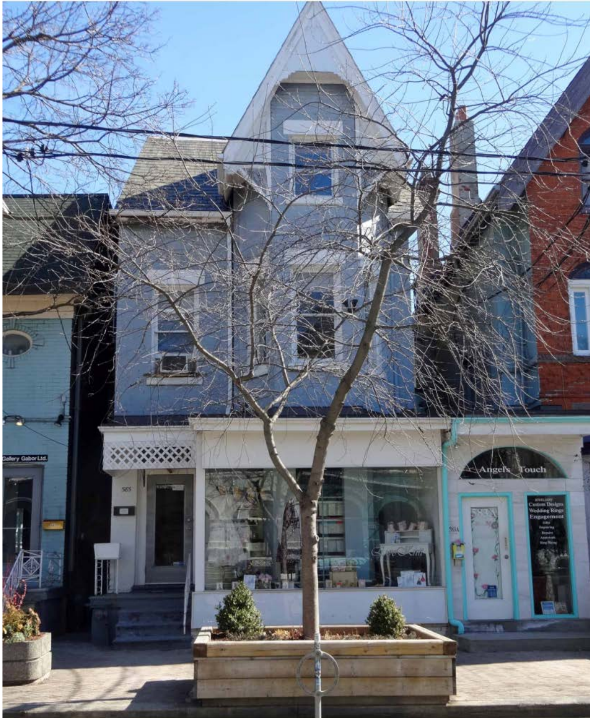
585 Markham Street: showing the west (principal) elevation (HPS, 2015)
