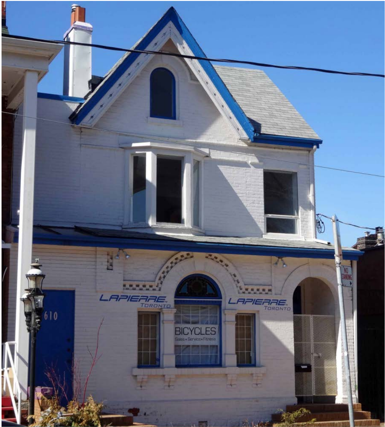
610 Markham Street: showing the east (primary) elevation (HPS, 2015)
