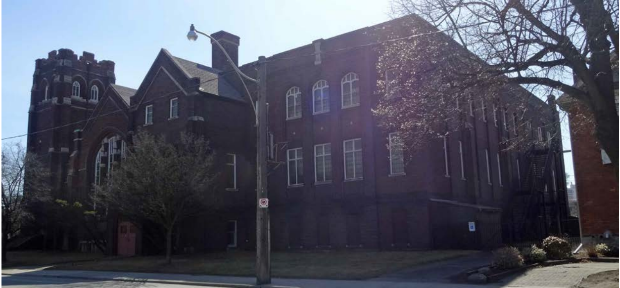
North and West Elevations - 260 High Park Avenue
