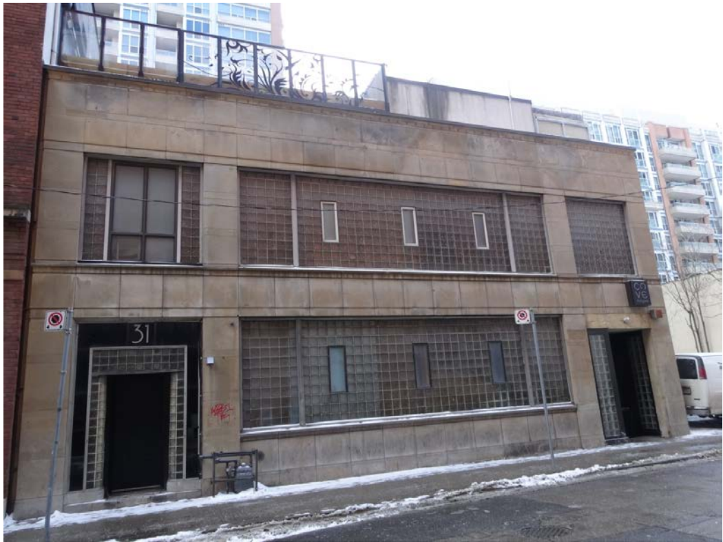
View of 31 Mercer Street- Pilkington Brothers Office Building - North Elevation
