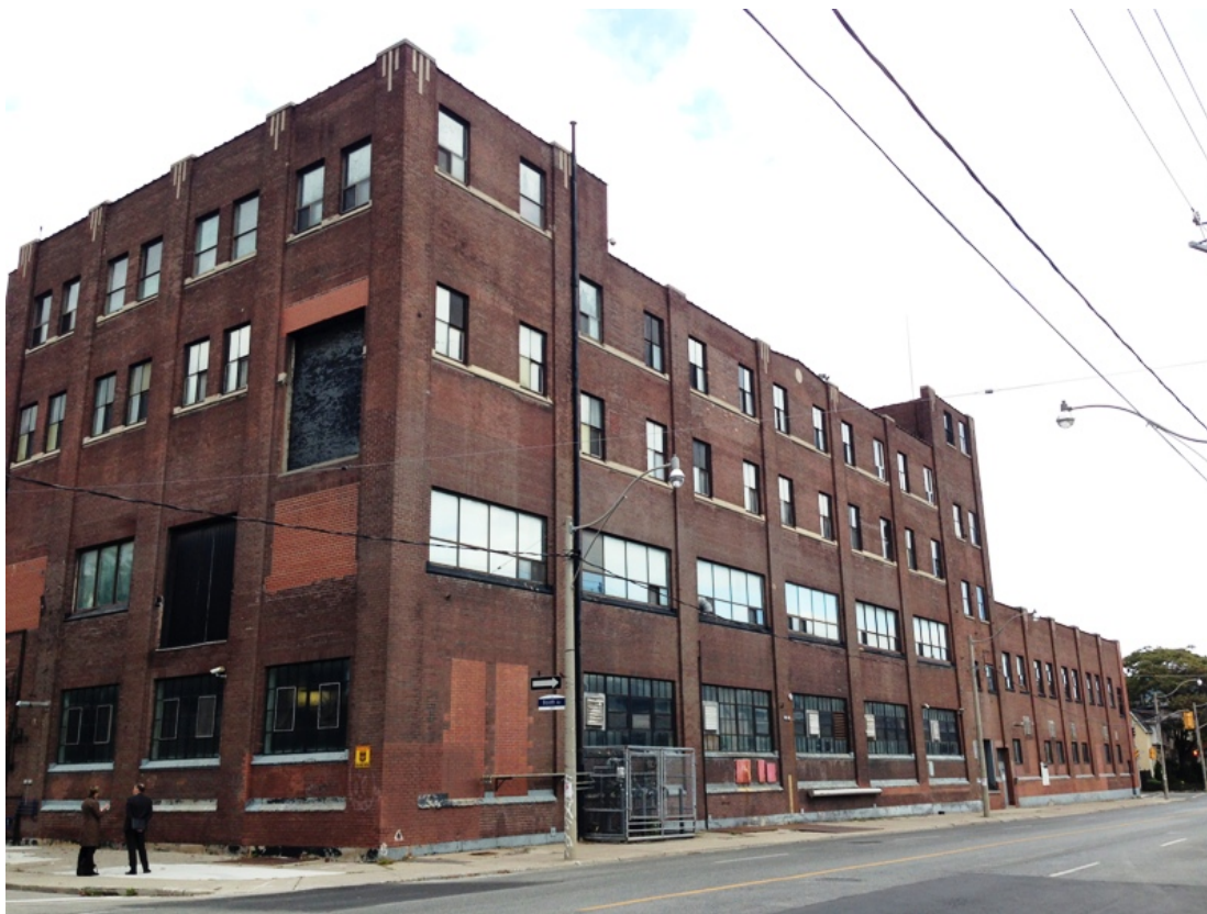
Photograph of the principal, south elevation on Eastern Avenue, and the side, west elevation facing Booth Avenue. (Heritage Preservation Services [HPS], 2016)
