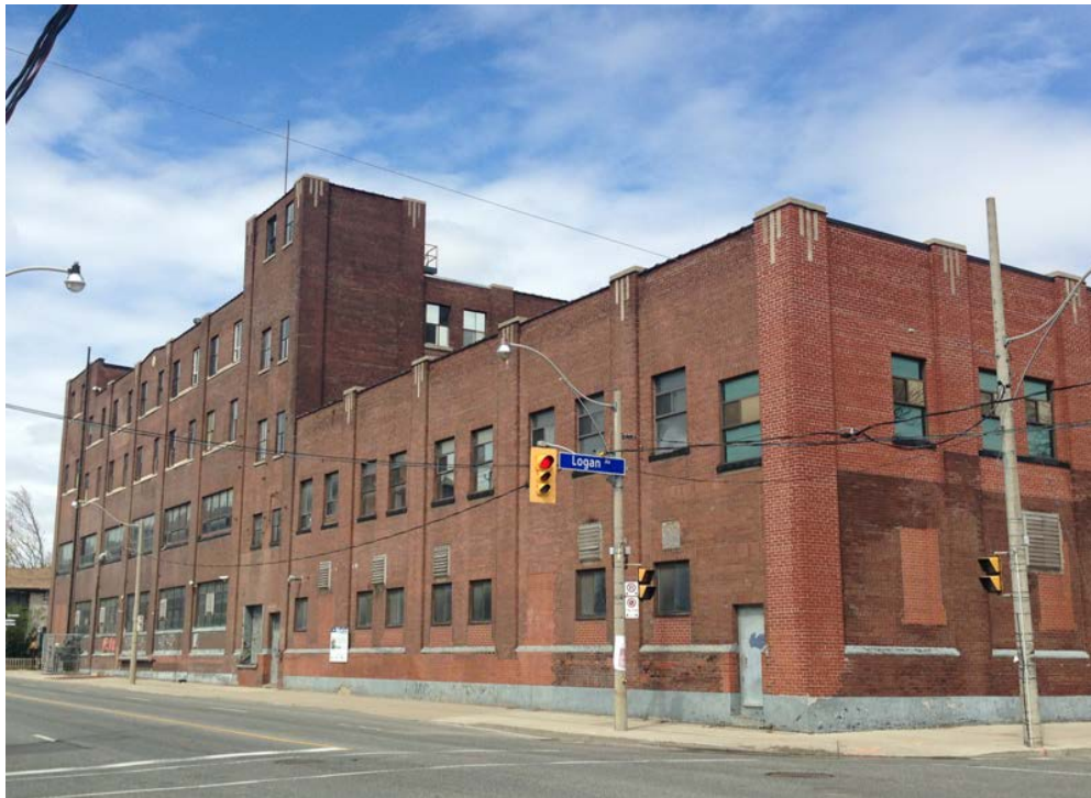
Photograph of the principal, south elevation on Eastern Avenue and a portion of the side, east elevation facing Logan Avenue (HPS, 2017)
