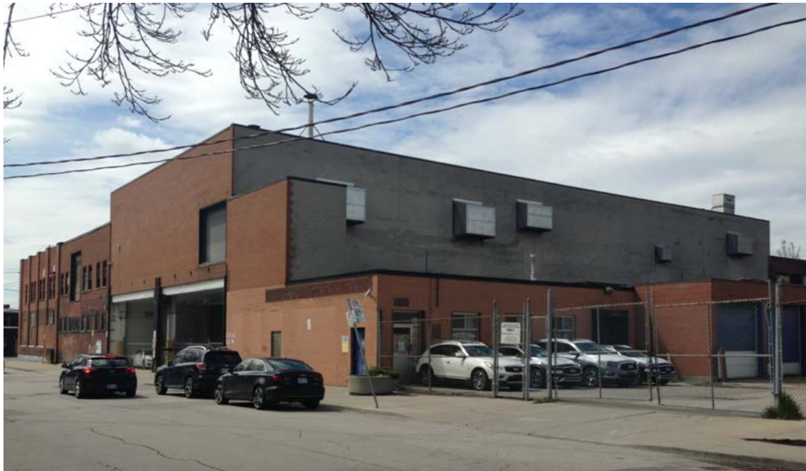
Photograph of the east and north elevations from Logan Avenue (HPS, 2017)
