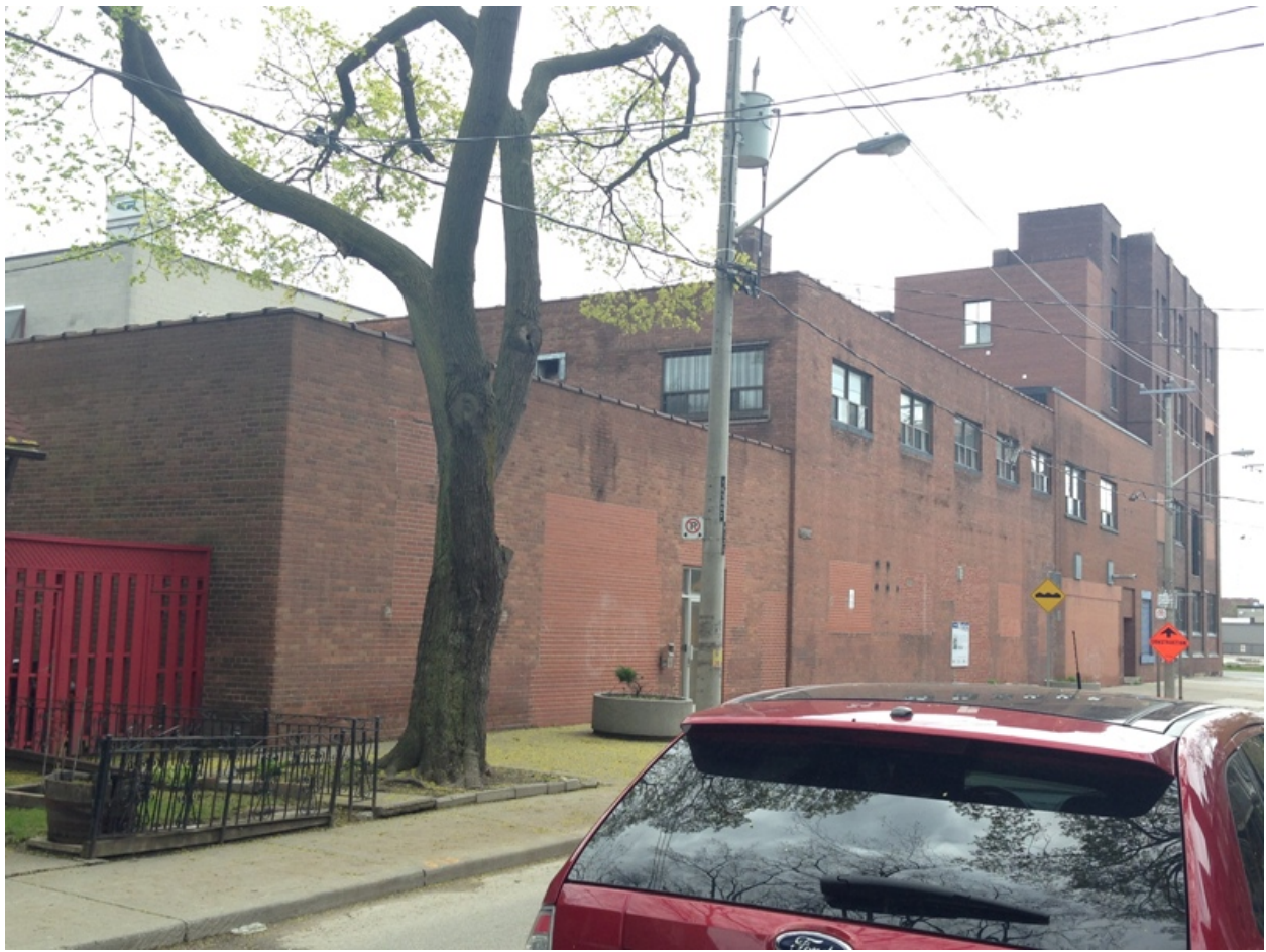
24. Side and north elevations as seen from Booth Avenue (HPS, 2017)
