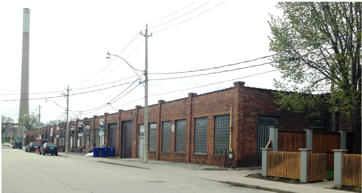
30. Industrial Building, west side, Logan Avenue, south of Eastern Avenue (HPS, 2017)
