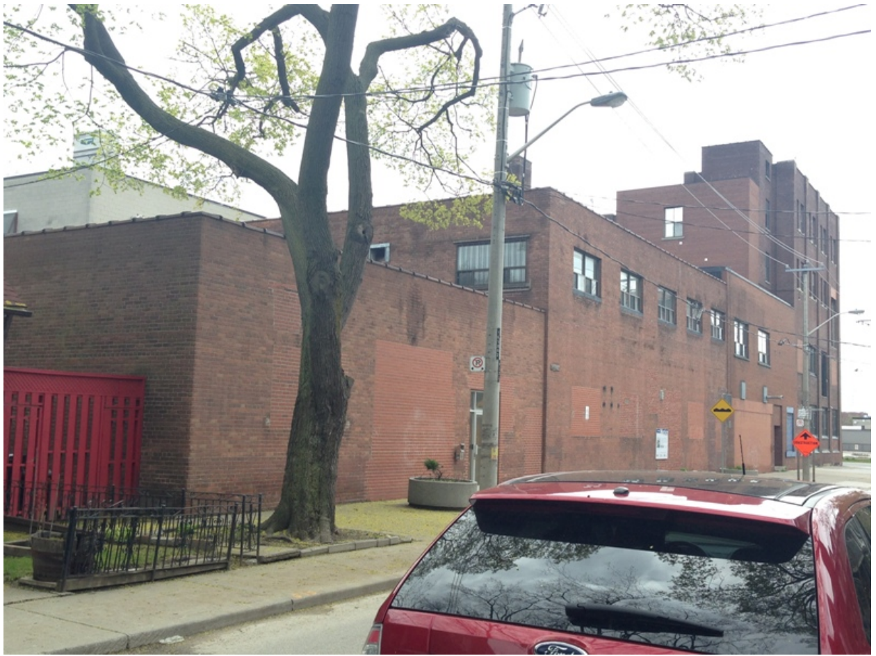
Photograph of the west and north elevations from Booth Avenue (HPS, 2017)
