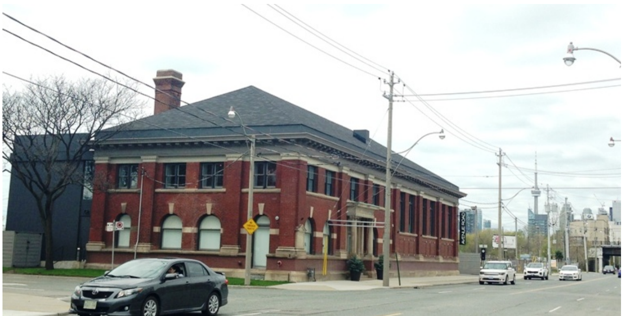
28. Consumers Gas, Station B, 415 Eastern Avenue (HPS, 2017)
