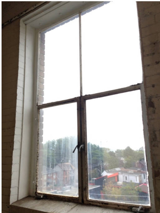
16. Interior view of metal windows installed with the 1926 additions to the complex, showing the opening bottom sections.
