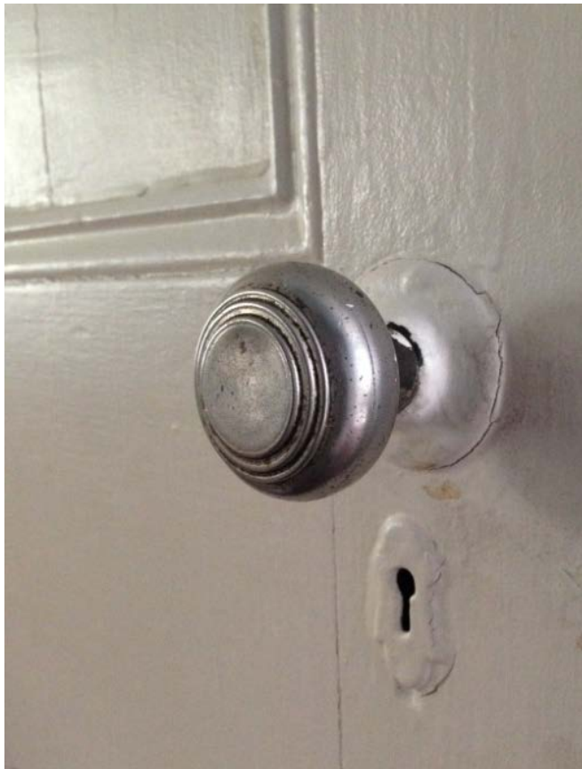
23. Typical door handle seen on exterior and interior doors and fielded panel moulding of door (HPS, 2017)
