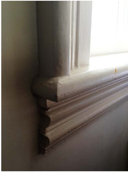
21. Living room window sill showing profile of mouldings (HPS, 2017)
