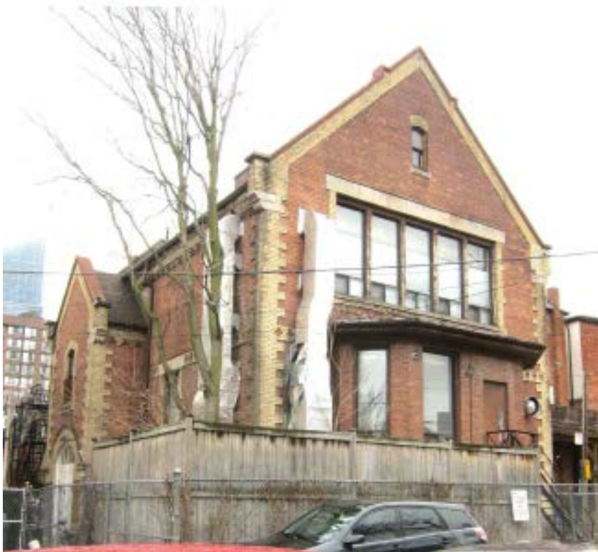
East elevation of the Allan School at 349 George Street.
