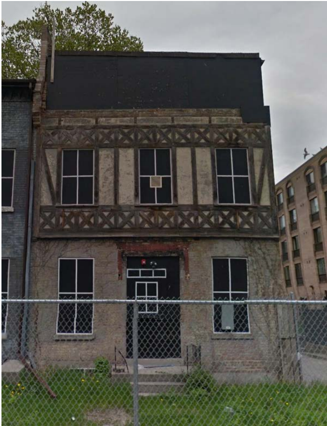
Fegan Boy's Home at 295 George Street after City stabilization work
