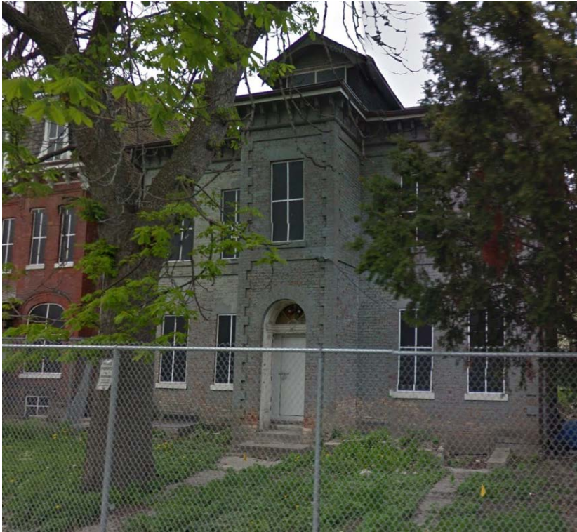
West elevation of Thomas Meredith House at 305 George Street.
