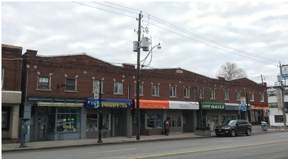
647A-669 Mount Pleasant Road (Heritage Preservation Services, 2017)
