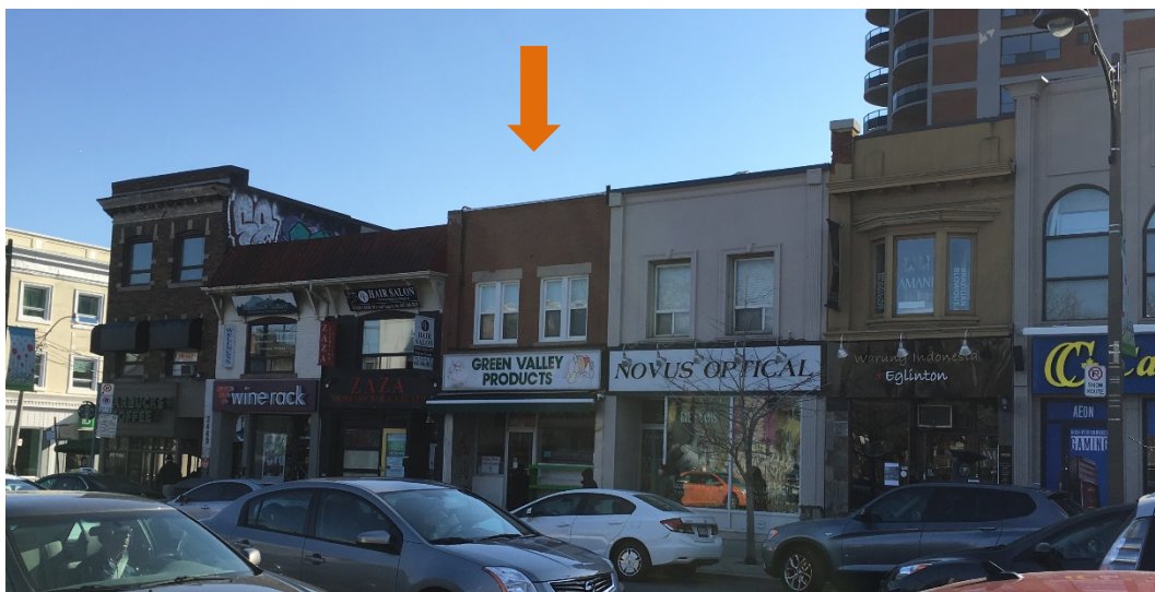
2443 Yonge Street (Heritage Preservation Services, 2017)
