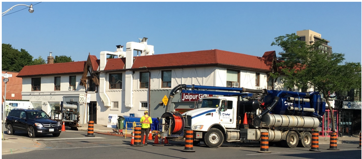
2066 Yonge Street (Heritage Preservation Services, 2017)
