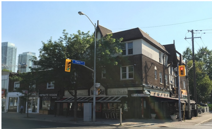
2075 Yonge Street (Heritage Preservation Services, 2017)
