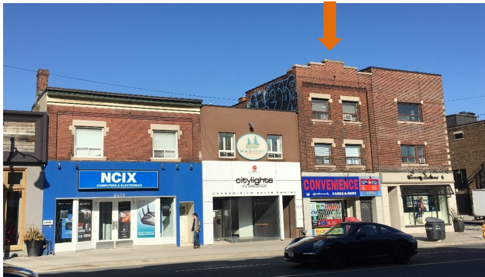
2482 Yonge Street (Heritage Preservation Services, 2017)
