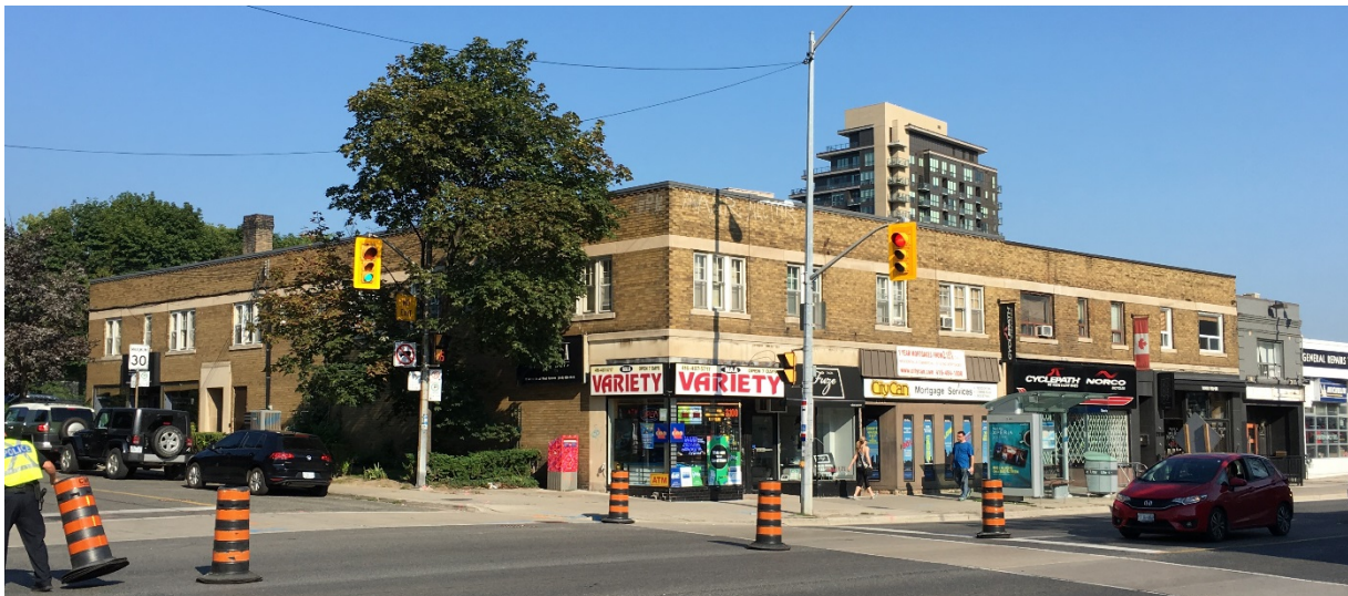
2100 Yonge Street (Heritage Preservation Services, 2017)
