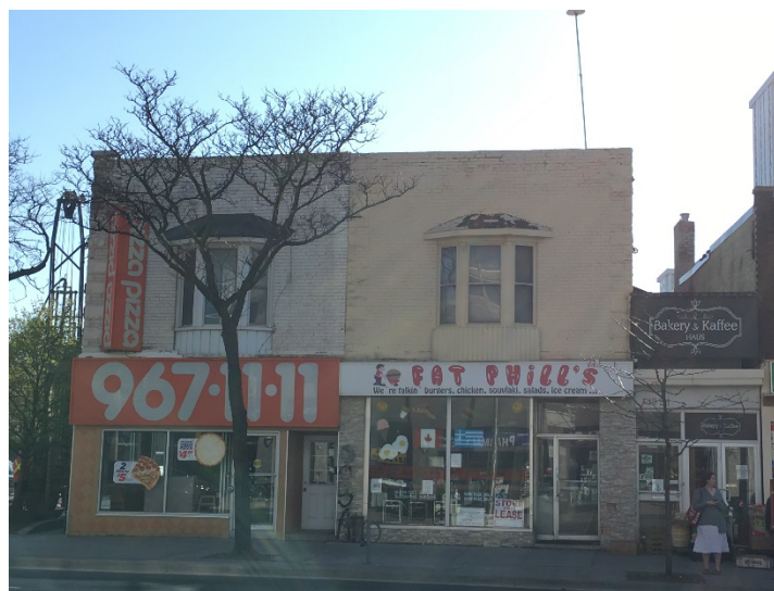
1919A and 1923 Yonge Street (Heritage Preservation Services, 2017)
