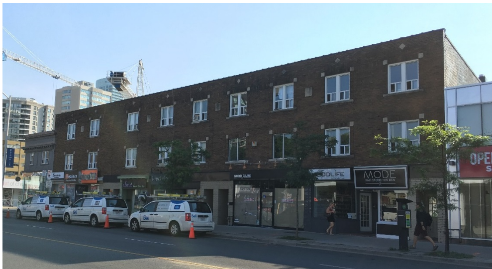
2093-2109 Yonge Street (Heritage Preservation Services, 2017)
