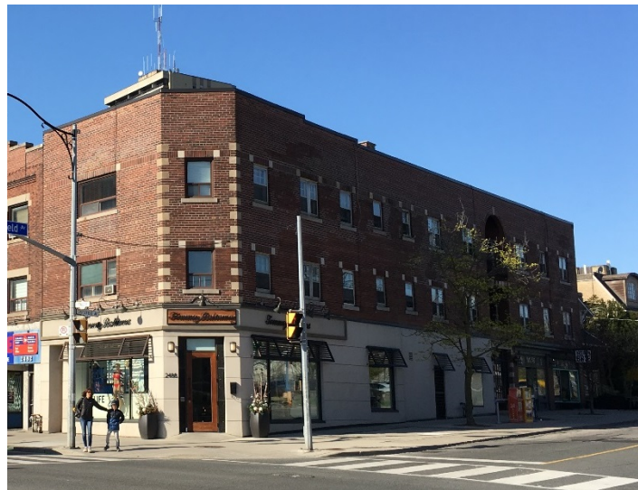
2488 Yonge Street (Heritage Preservation Services, 2017)
