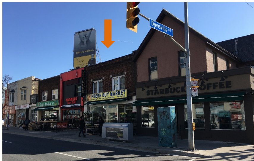
1913 Yonge Street (Heritage Preservation Services, 2017)
