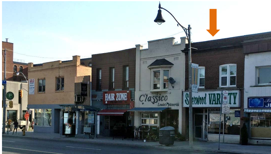
2547 Yonge Street (Heritage Preservation Services, 2017)
