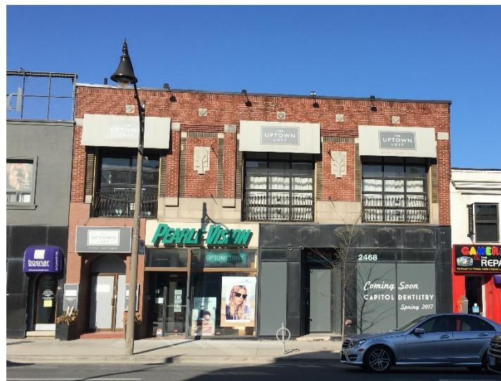
2468 Yonge Street (Heritage Preservation Services, 2017)
