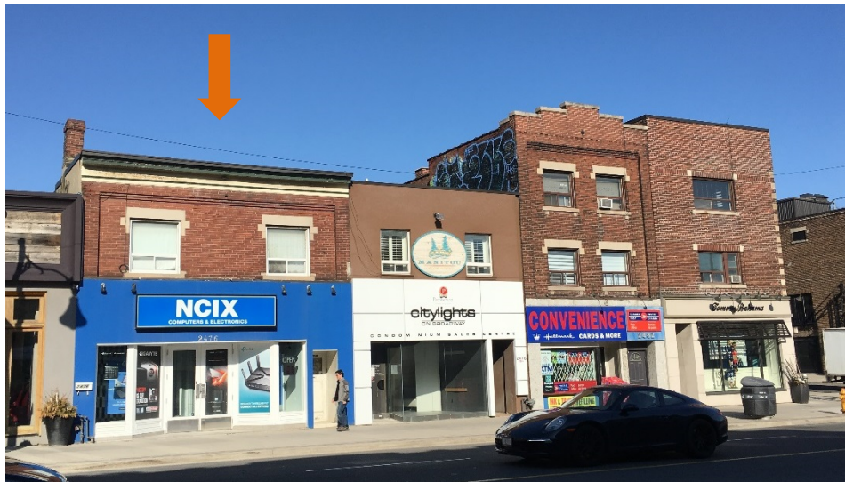
2476 Yonge Street (Heritage Preservation Services, 2017)
