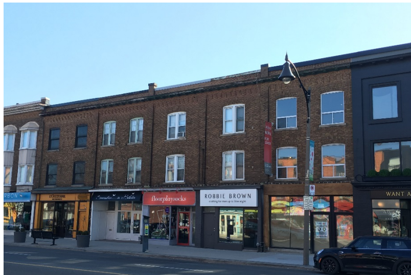
2581-2589 Yonge Street (Heritage Preservation Services, 2017)
