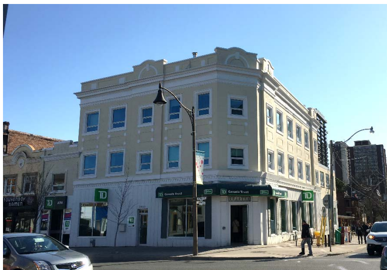
2453 Yonge Street (Heritage Preservation Services, 2017)
