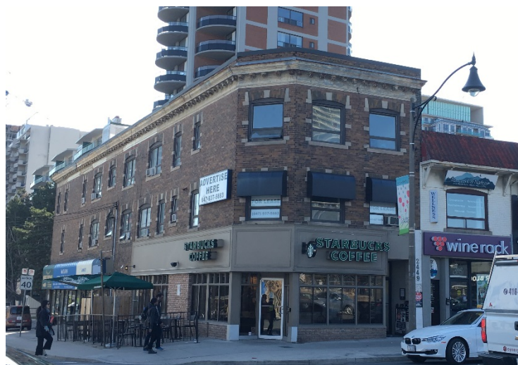
2449 Yonge Street (Heritage Preservation Services, 2017)
