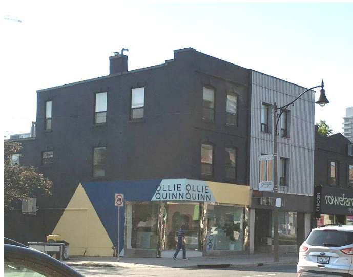
2507-2509 Yonge Street (Heritage Preservation Services, 2017)
