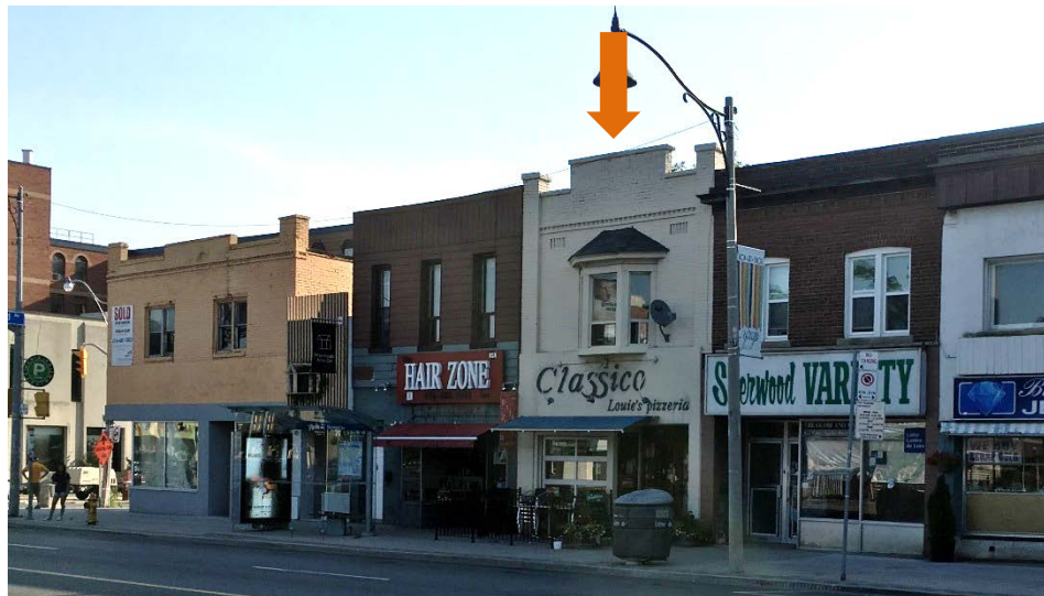
2549 Yonge Street (Heritage Preservation Services, 2017)
