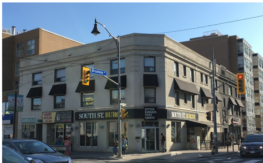
2383 Yonge Street (Heritage Preservation Services, 2017)
