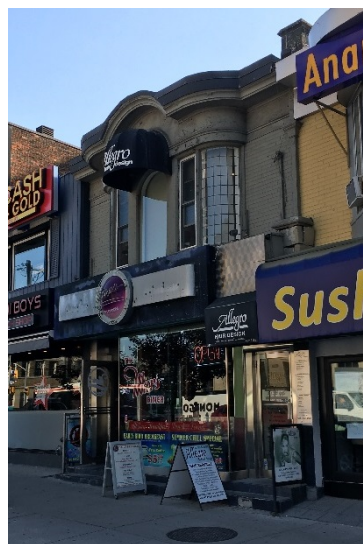
2363 Yonge Street (Heritage Preservation Services, 2017)
