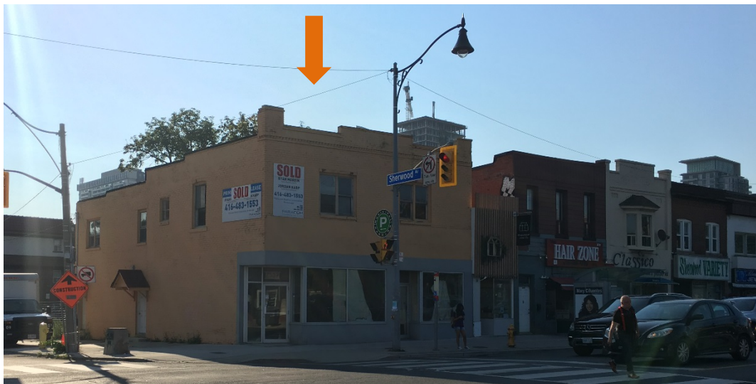
2555 Yonge Street (Heritage Preservation Services, 2017)
