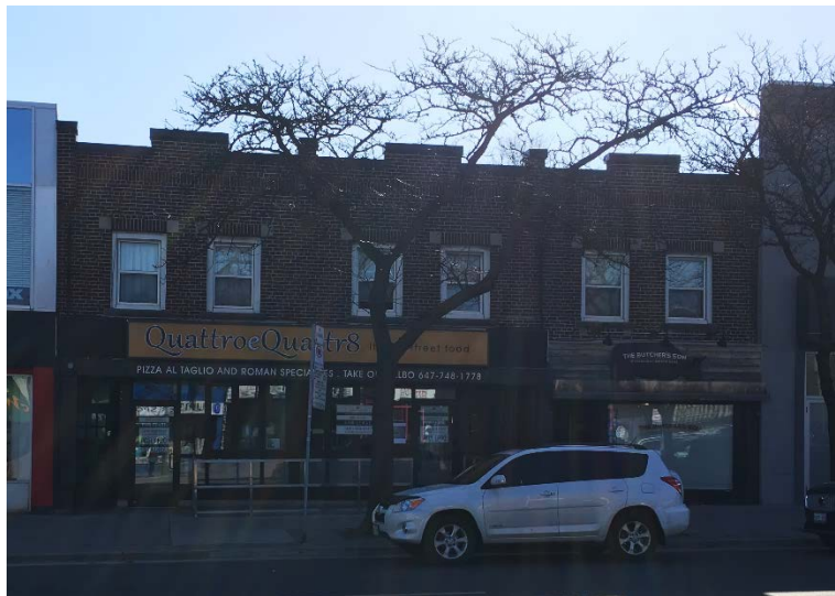
2055-2059 Yonge Street (Heritage Preservation Services, 2017)
