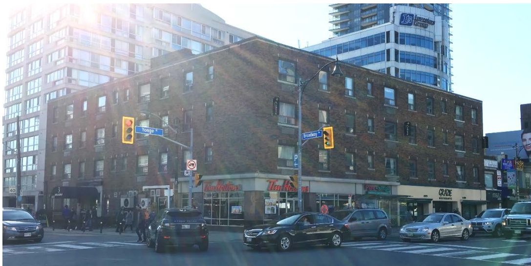
2377 Yonge Street (Heritage Preservation Services, 2017)
