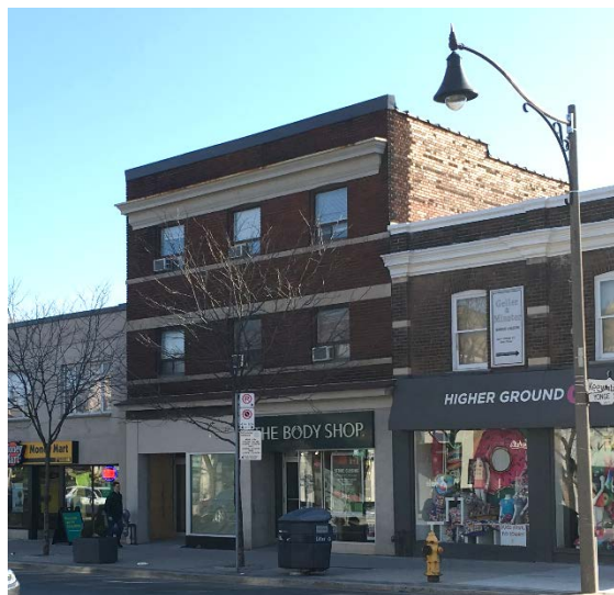
2515 Yonge Street (Heritage Preservation Services, 2017)
