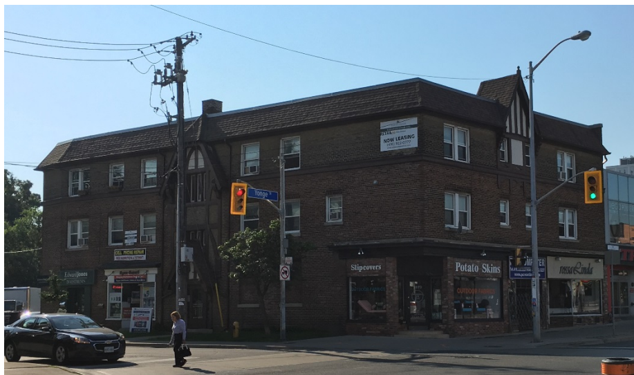
2069 Yonge Street (Heritage Preservation Services, 2017)
