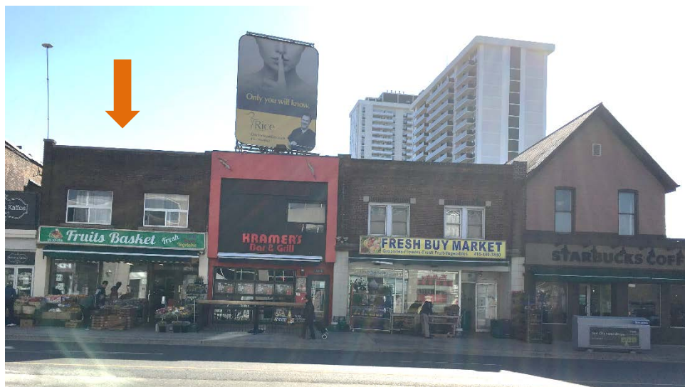
1919 Yonge Street (Heritage Preservation Services, 2017)
