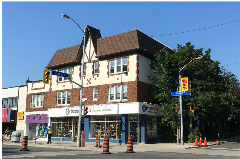
2094 Yonge Street (Heritage Preservation Services, 2017)
