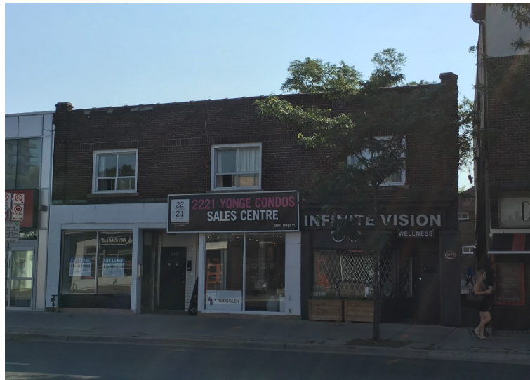
2079-2085 Yonge Street (Heritage Preservation Services, 2017)
