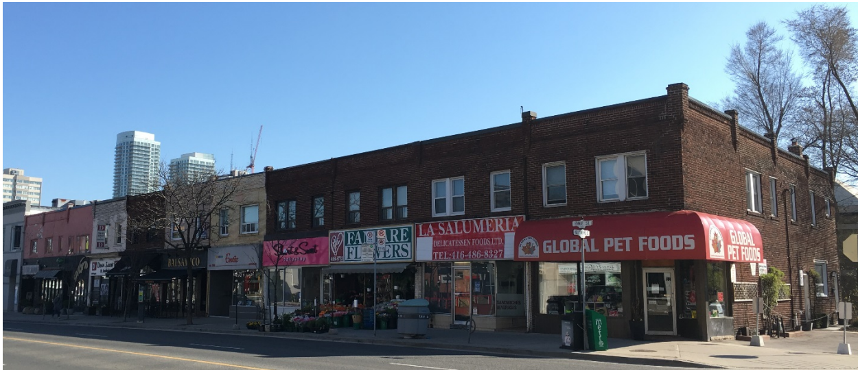
2019-2039 Yonge Street (Heritage Preservation Services, 2017)
