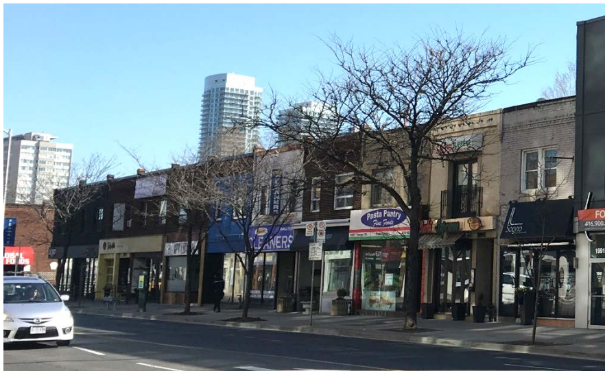
1997-2013 Yonge Street (Heritage Preservation Services, 2017)
