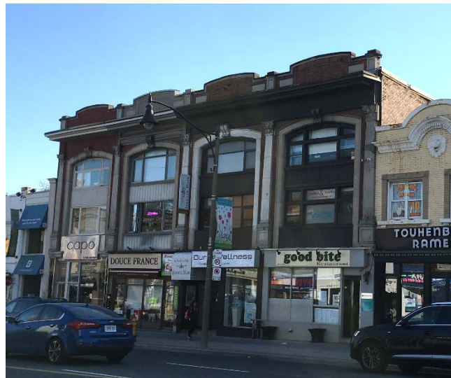
2463-2473 Yonge Street (Heritage Preservation Services, 2017)
