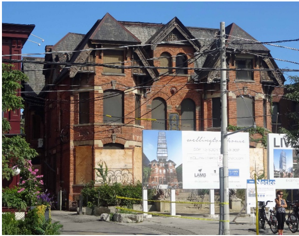
4a. Current Photograph, principal (south) elevation
