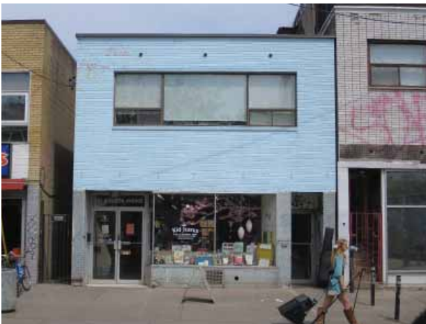
FIG. 7-14 COMMERCIAL VERNACULAR, POSTWAR, AUGUSTA AVENUE (THA 2016).
