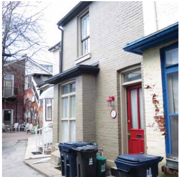
FIG. 2-10 WORKER COTTAGES IN FITZROY TERRACE (THA 2016).
