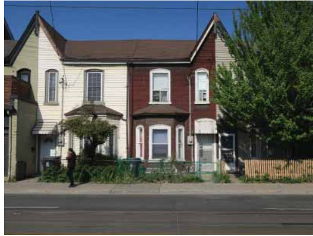
FIG. 7-8 RESIDENTIAL VERNACULAR VICTORIAN, BATHURST STREET (THA 2016).
