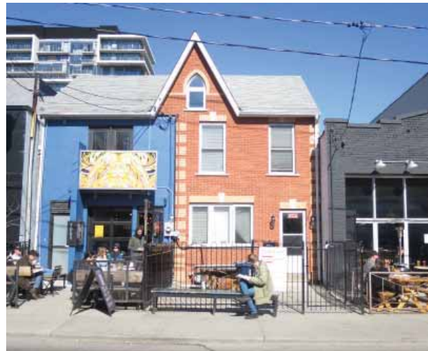
FIG. 5-1 A FIELD SURVEYOR SITS RECORDING A BUILDING IN THE STUDY AREA, AUGUSTA AVENUE (THA 2016).
