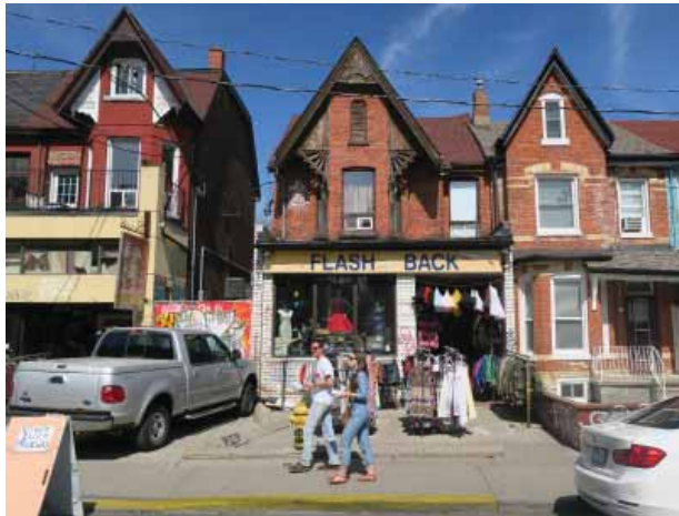
FIG. 7-25 STOREFRONT ADDITIONS, KENSINGTON AVENUE (THA 2016).
