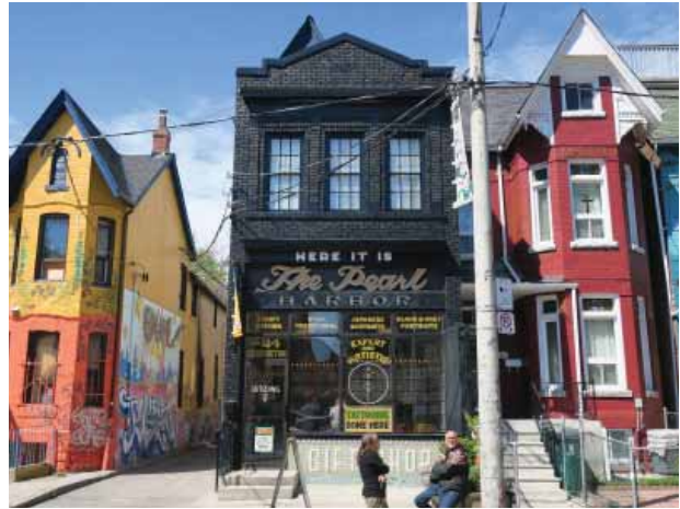
FIG. 7-26 STOREFRONT ADDITIONS, KENSINGTON AVENUE (THA 2016).
