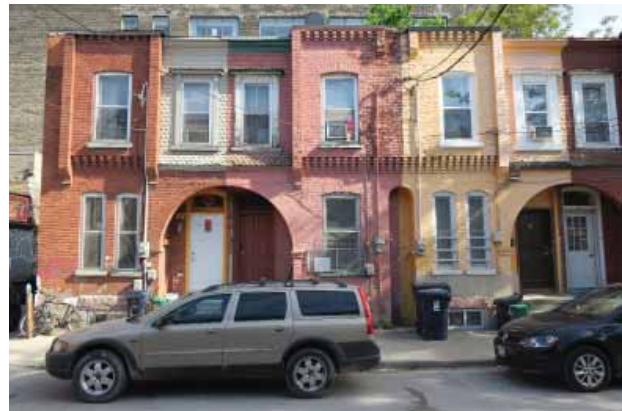
FIG. 2-9 WORKER COTTAGES IN GLEN BAILLIE PLACE (THA 2016).
